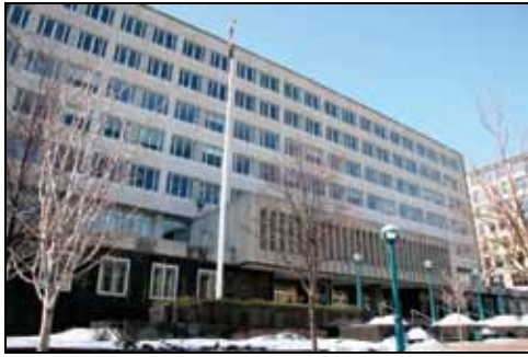
Central District Station/Administrative Offices
