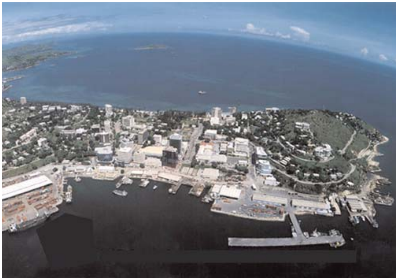
Port Moresby—Main Wharf facing SE
