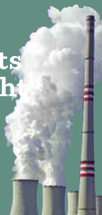
image COAL FIRED POWER PLANT. © F. FOX/DREAMSTIME
