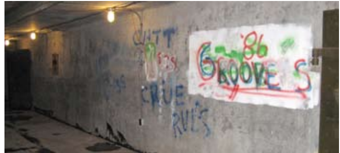
Main corridor wall before cleaning
