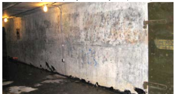
Corridor wall after cleaning.
