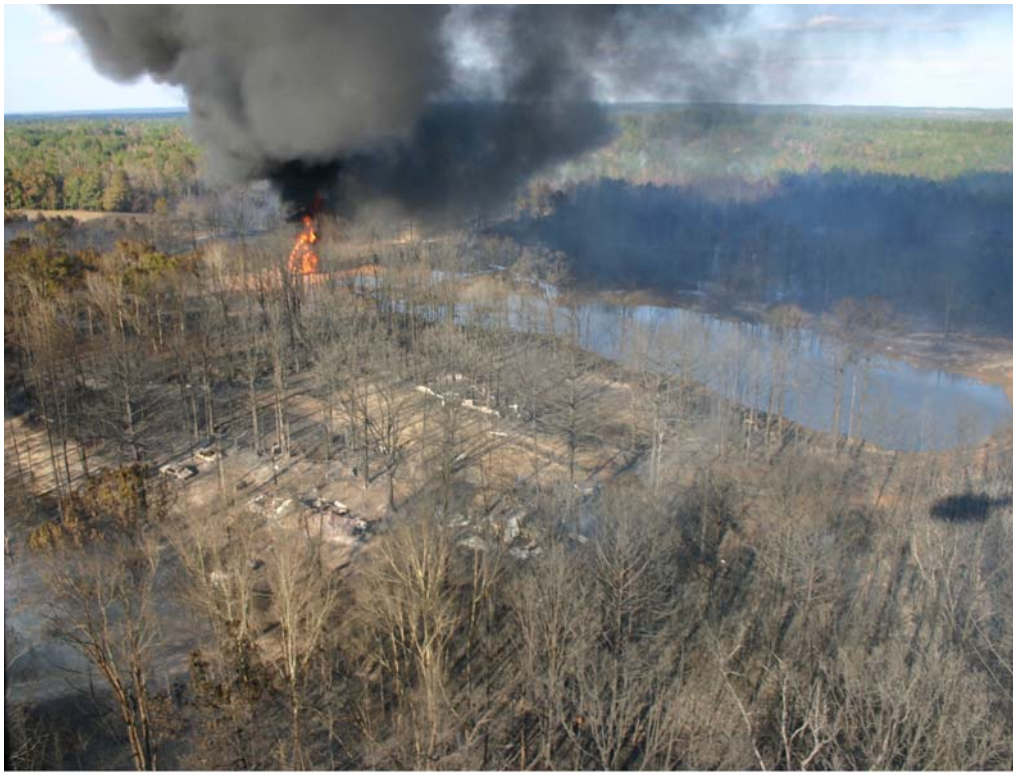
Figure 2. Aerial view of fire from pipeline rupture showing nearby destroyed houses.
