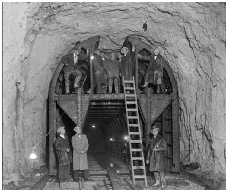
Clay exposed in the yet unlined walls of the Chicago Avenue water tunnel (1928; DN-0086862, Chicago Daily News negatives collection, Chicago Historical Society).
