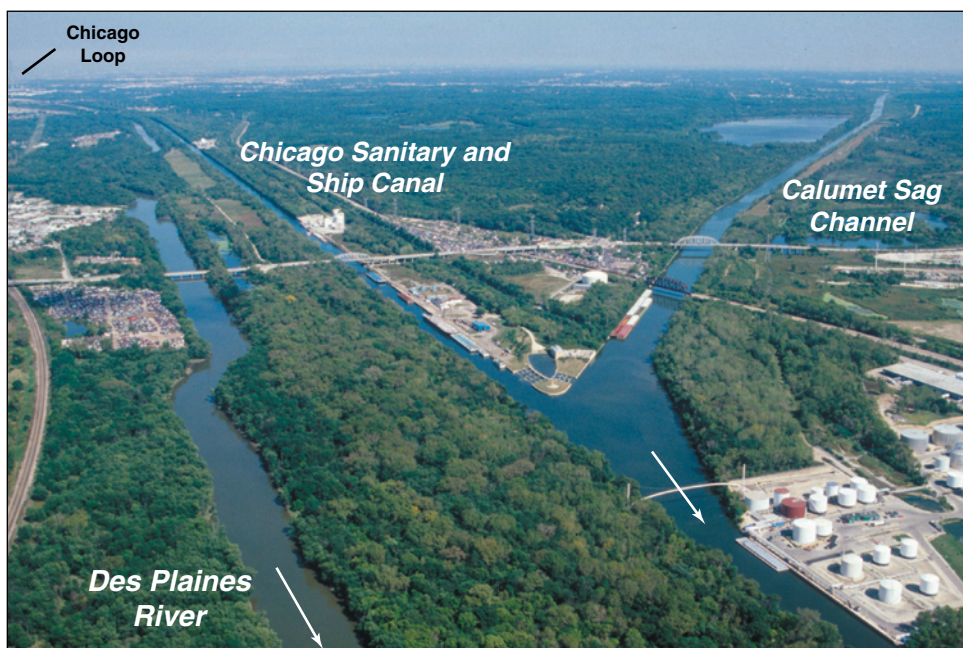
View looking east showing the three waterways that flow through the Chicago Outlet Valley (Sept 2002; photo by M. Chrzastowski, ISGS).
