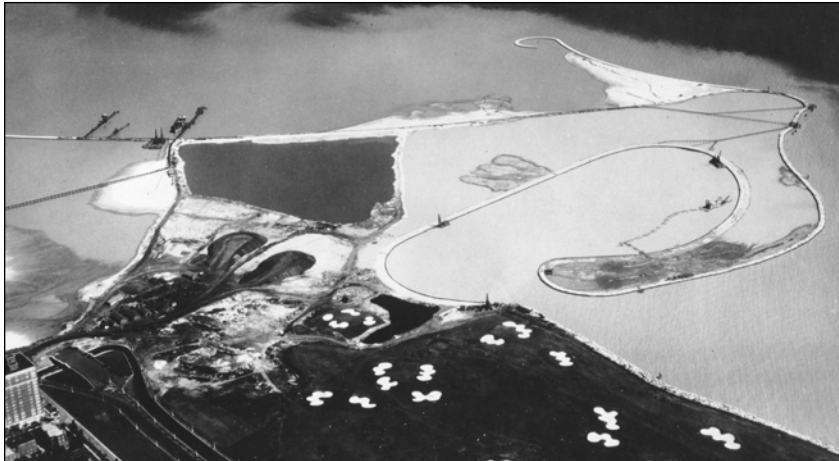
This aerial photo from September 1931 shows the ongoing construction of Montrose Peninsula. Waveland Golf Course is in the foreground. The discharge of fill sand has produced a plume of suspended sediment that clouds the nearshore area (photo courtesy of Great Lakes Dredge and Dock Co., Oakbrook, Illinois).
