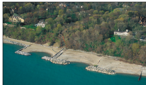
Example of beach cells built along private lakeshore in Lake Forest (May 3, 2000; photo by M. Chrzastowski, ISGS).
