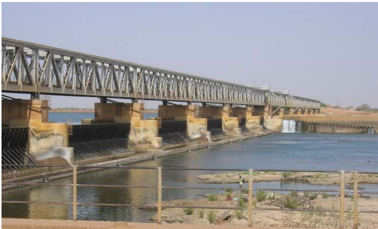
Markala barrage in the Niger river near Ségou at the downstream side – used for irrigation of the irrigation zone of the Office du Niger.
