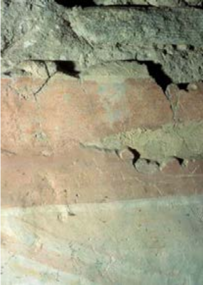
Detail showing the lack of contact between the wooden beam and fresco layers
