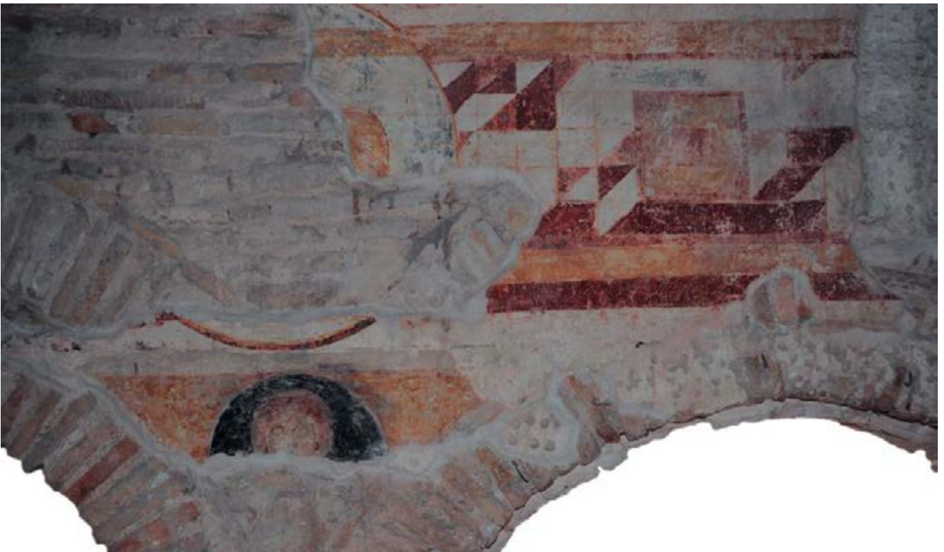
San Salvatore, detail of the southern wall of northern nave
