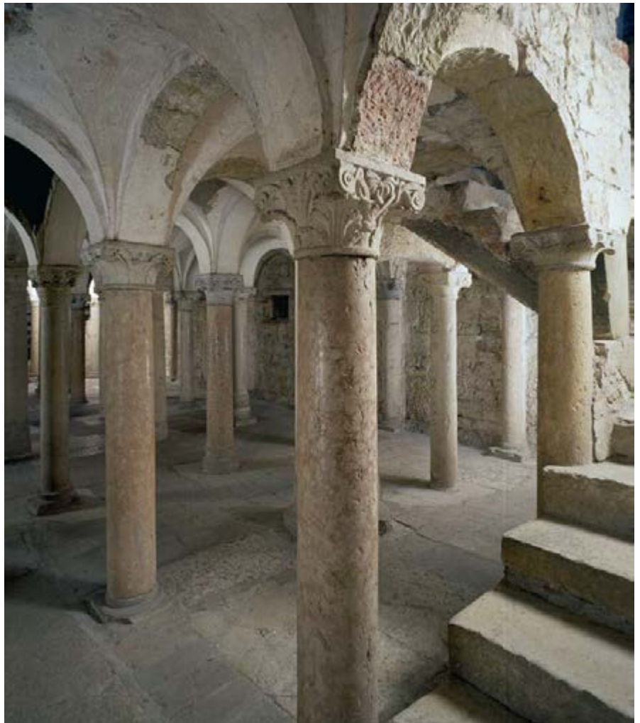
Romanesque widening of the crypt of San Salvatore
