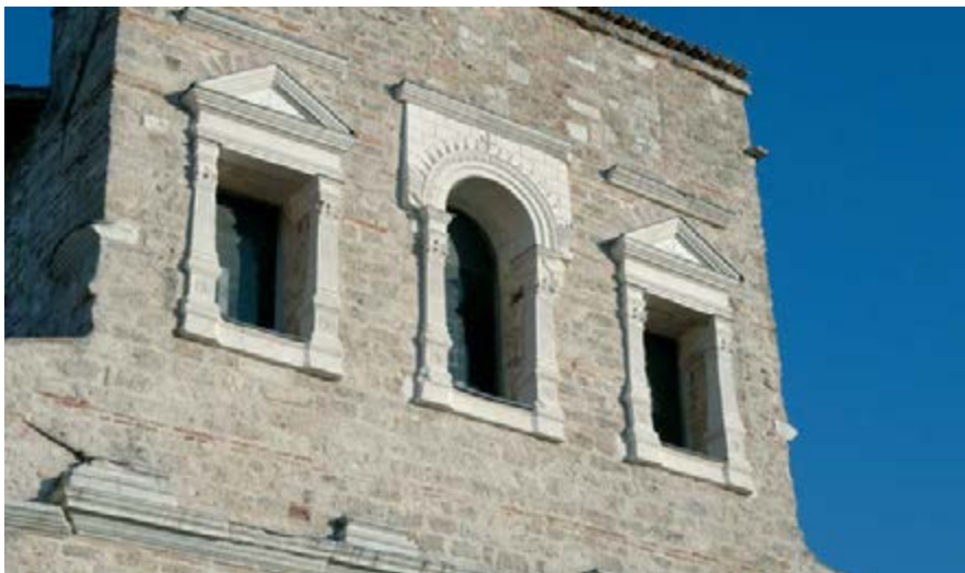
San Salvatore, façade. Detail of the windows
