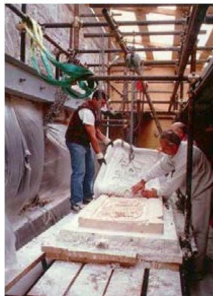
Mould of the church's main doorway (90s)
