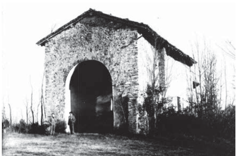
Santa Maria foris portas before the conservation interventions
