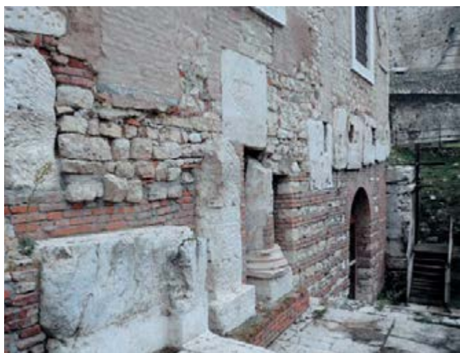
Remains of the Roman Theatre, re-used in Palazzo Maggi Gambara's foundations
