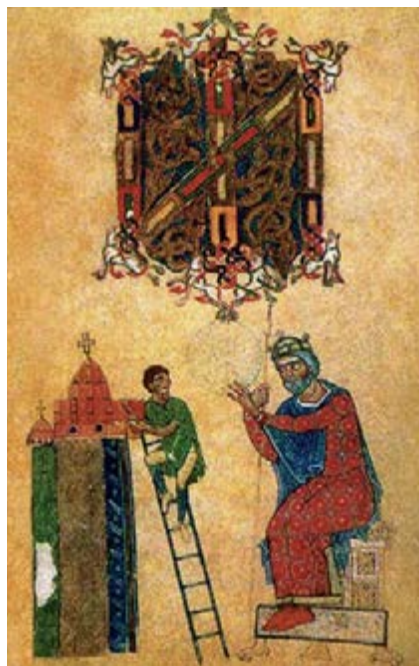
Duke Arechi II presides over the construction of the Church
