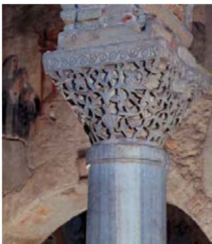
San Salvatore, one of the two "bread basket" style capitals of Byzantine origin, re-used in colonnade
