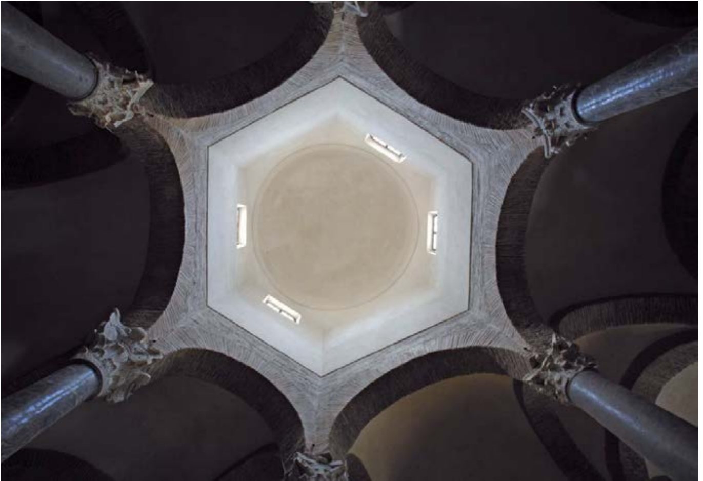
The central dome of vaulted system
