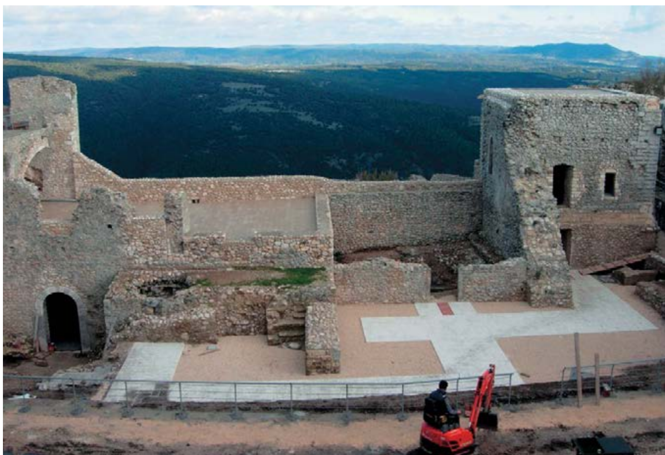
Conservation works at the Castle included in the buffer zone
