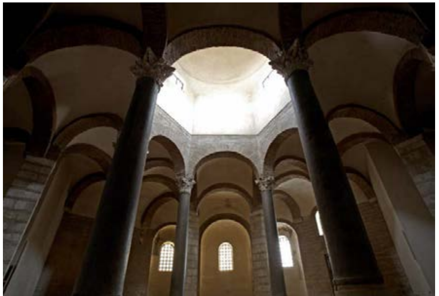
The Santa Sofia Church, vaults
