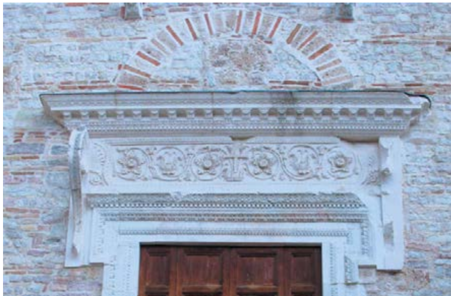
San Salvatore, main portal
