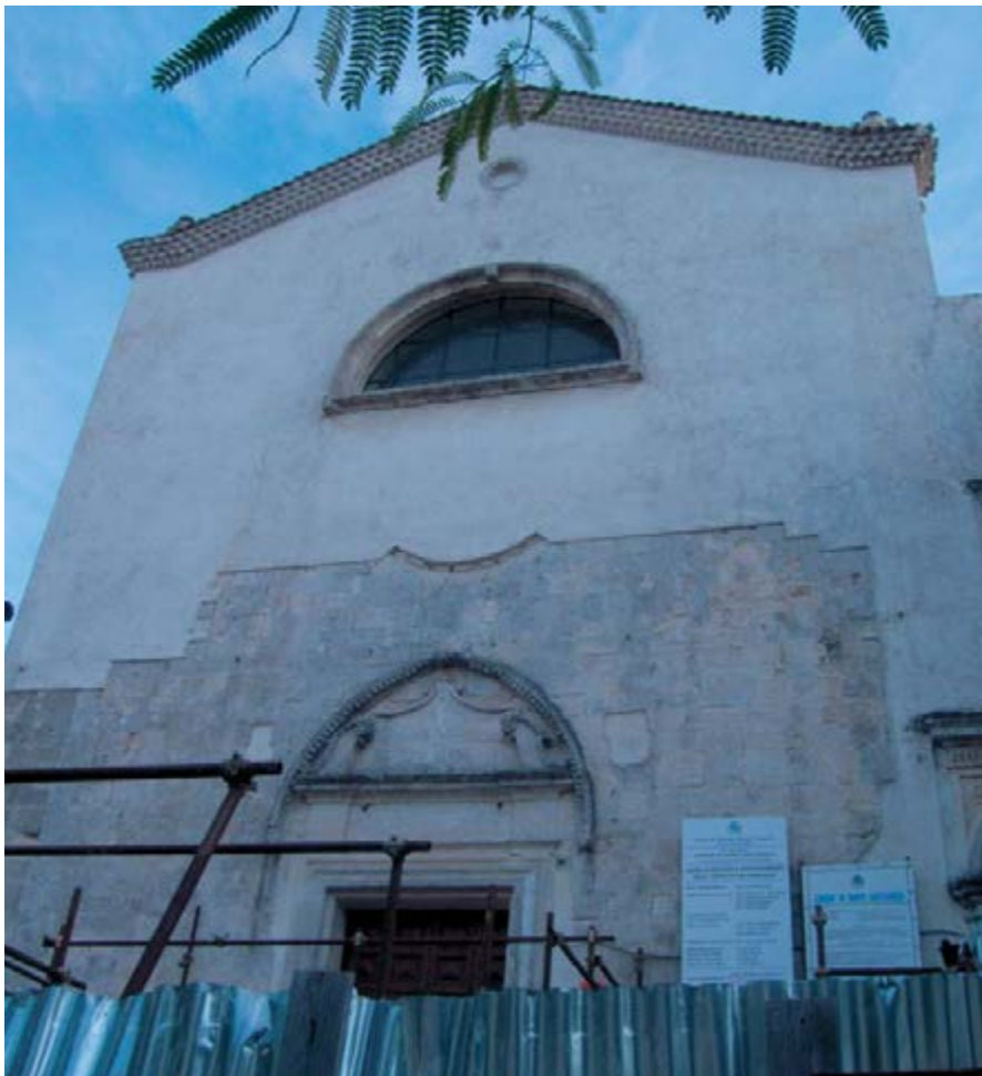
Conservation works on San Francesco complex
