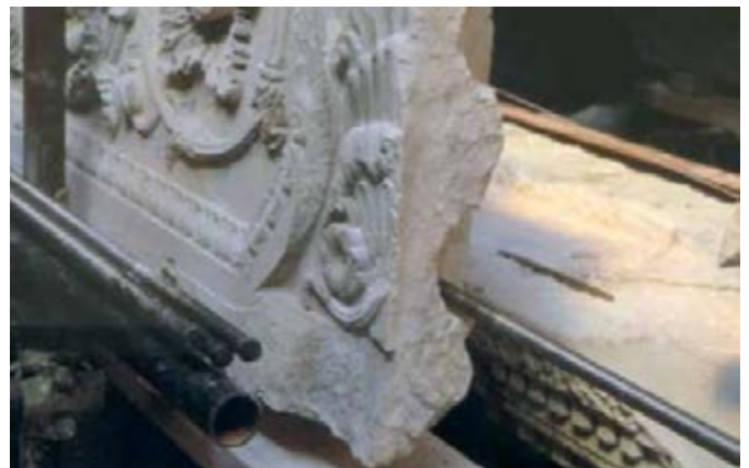
Main portal's architrave. Disassembly (90s)
