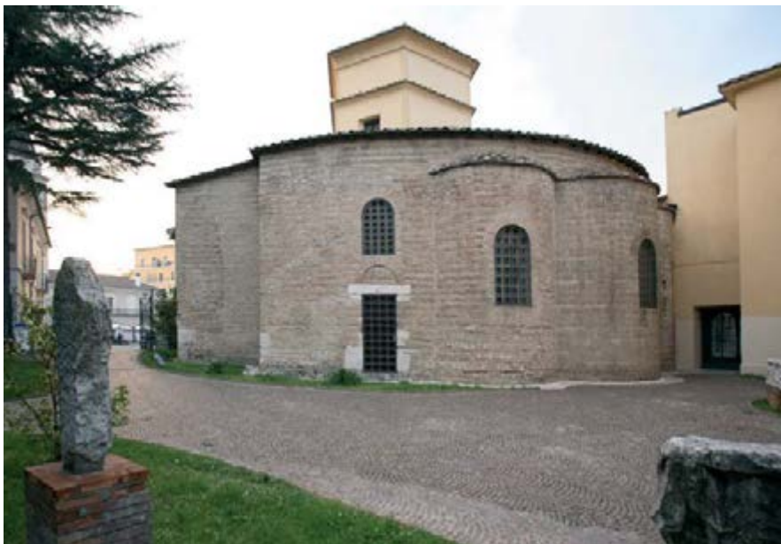
External view apses' side
