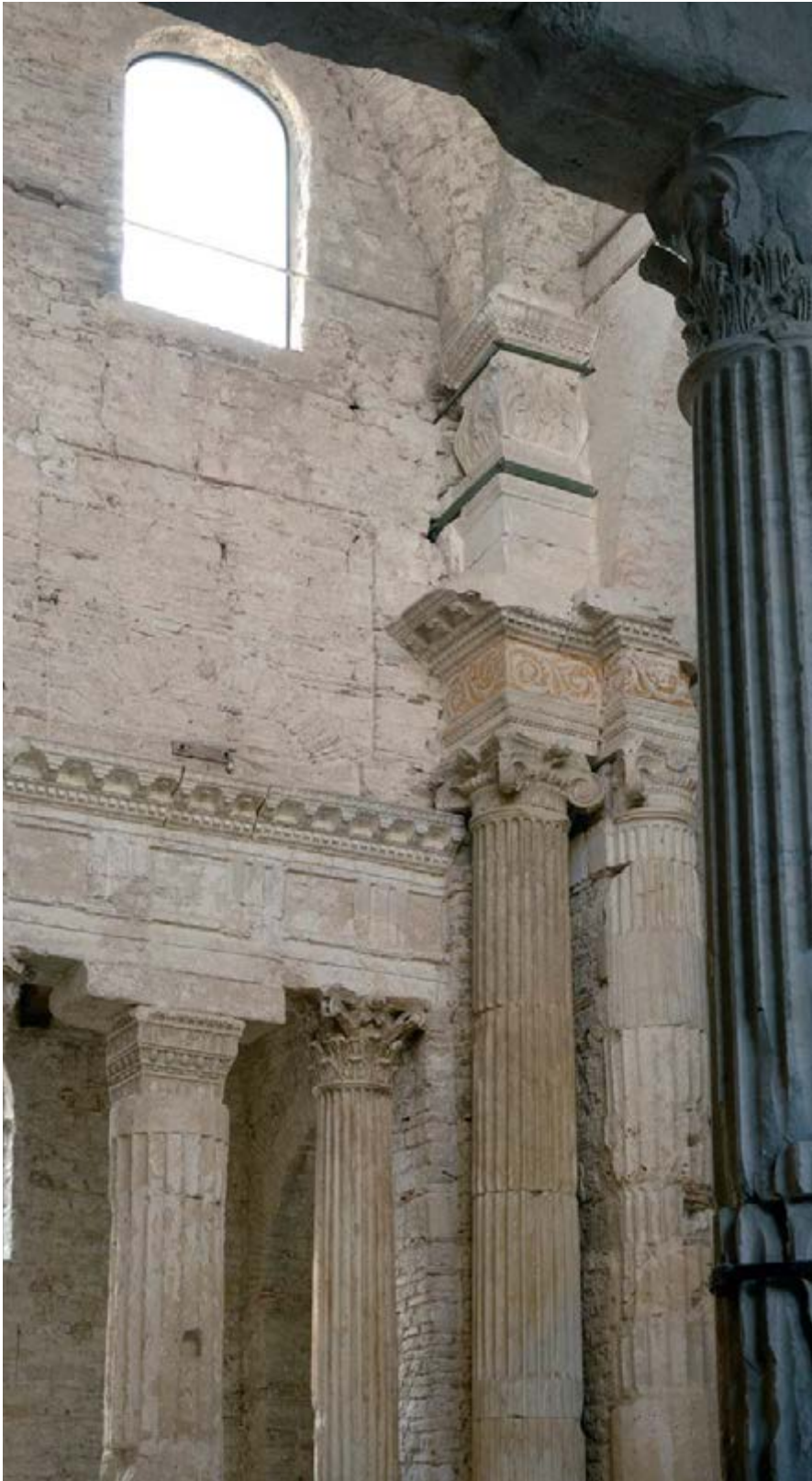
San Salvatore, presbytery. Detail of angular columns
