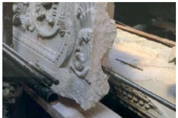
Main portal's architrave. Disassembly (90s)
