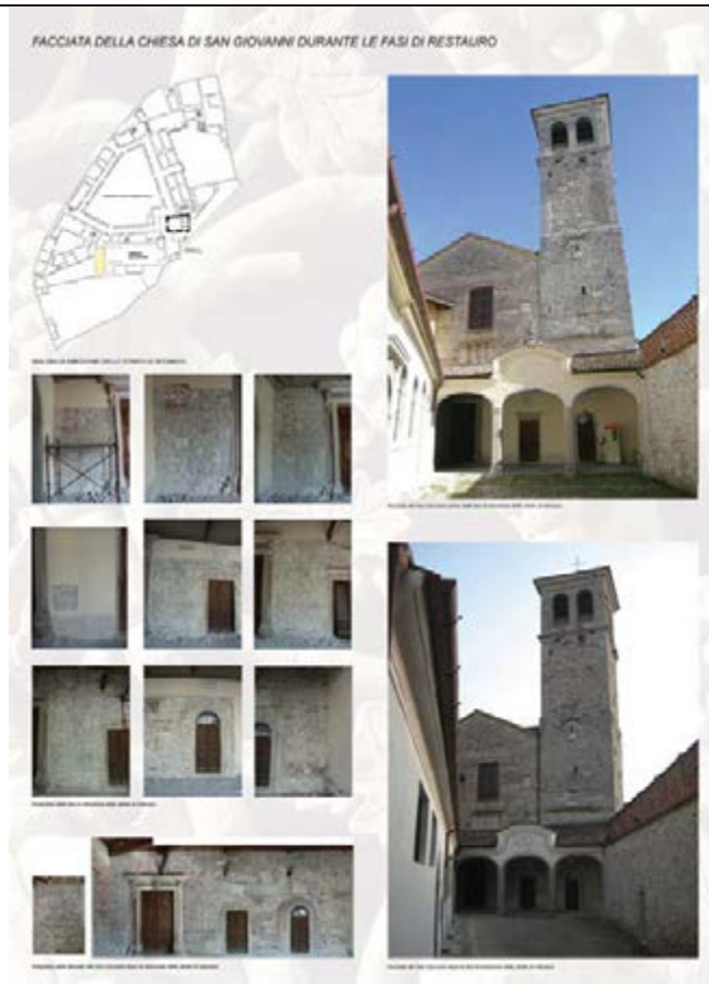
Restoration phases of the façade of the Church of S.Giovanni
