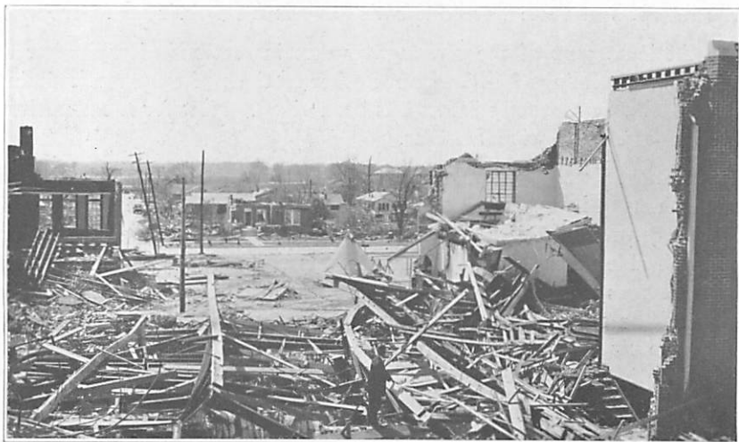
Figure 13.—The wreckage of the west wall and roof was thrown across the seats of the auditorium of the High School by the tornado of April 5, 1936.--Photographed toward the west, April 13, 1936.
