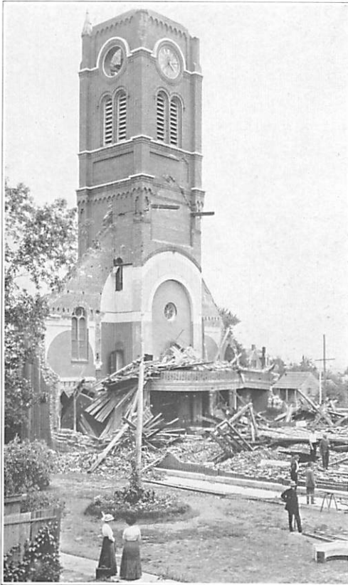
Figure 7.—The tower of Borrromeo Church, St. Charles, Mo., scarcely lost a brick in the tornado of July 7, 1915.--Photographed July 9, 1915.
