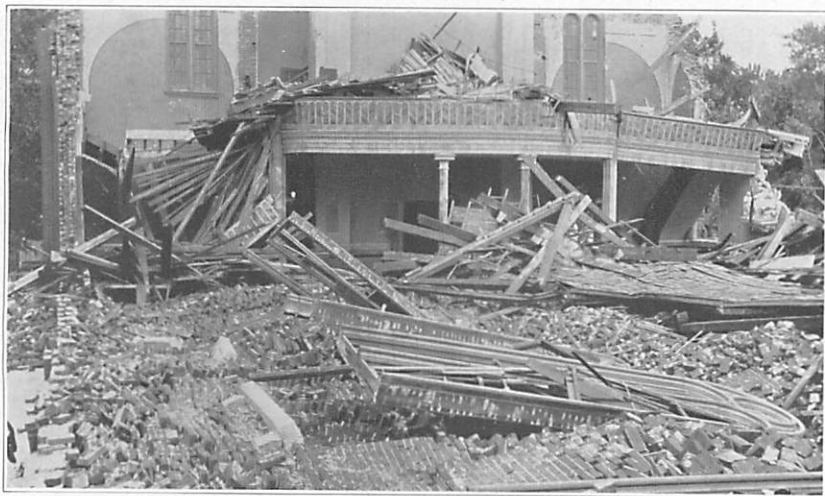
Figure 6.—The west wall of Borrromeo Church, St. Charles, Mo., which was blown across the pews by the tornado of July 7, 1915. --Photographed July 9, 1915.
