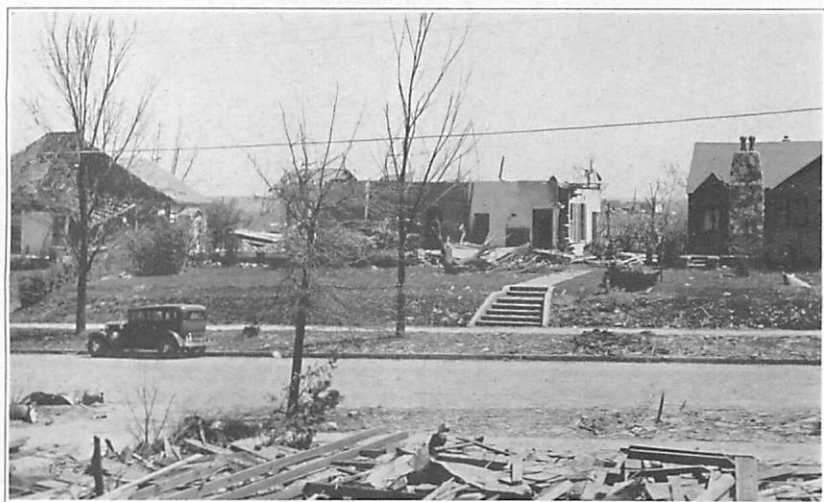
Figure 17.—This frame house on the north side of the Carnaggio house almost completely collapsed in the tornado of April 5, 1936 --Photographed April 13, 1936.
