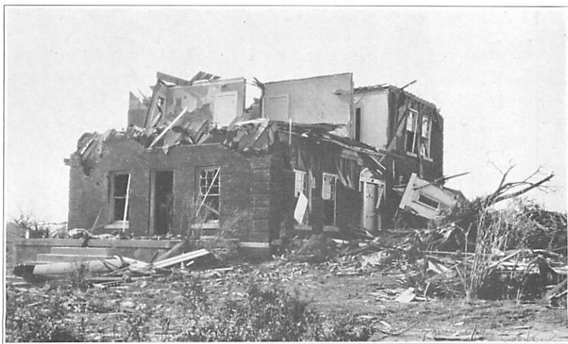
Figure 20.—This next door house, a brick veneer, was not completely blown away in the tornado of April 5, 1936, as the Huffman house was, but it is largely a wreck when compared with the Carnaggio house. Mortar so inferior as to crumble in the fingers is probably the chief reason.--Photographed April 13, 1936.
