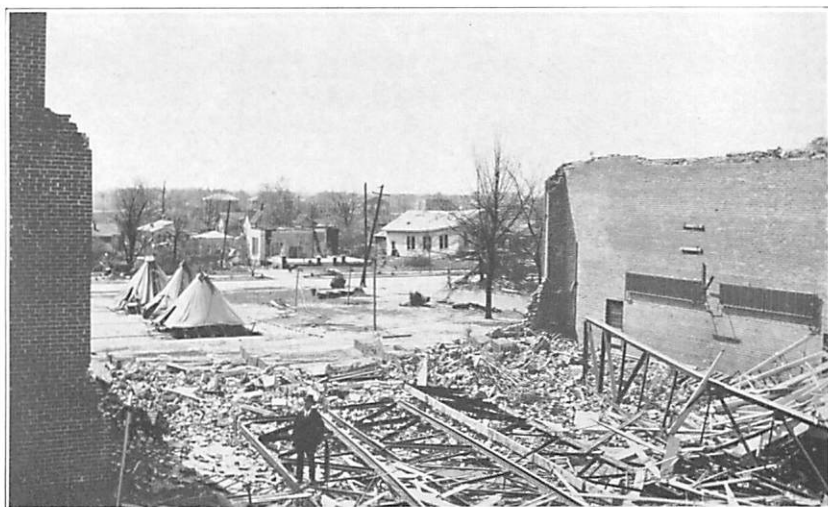
Figure 14.—In a like manner the wreckage of the west wall and the roof was thrown across the floor of the gymnasium of the High School by the tornado of April 5, 1936.--Photographed toward the west, April 13, 1936.
