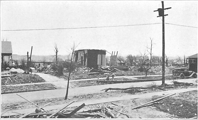
Figure 18.—This frame house on the south side of the Carnaggio house likewise almost completely collapsed in the tornado of April 5, 1936.--Photographed April 13, 1936.
