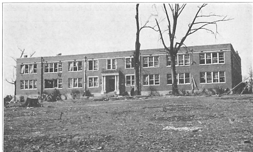
Figure 15.—The windows and drain pipes of the south front of the High School were badly battered by flying wreckage as were the trunks and the limbs of these two trees, but this part of the building, and the east wing as well, scarcely lost a brick in the tornado of April 5, 1936.--Photographed toward the north, April 13, 1936.
