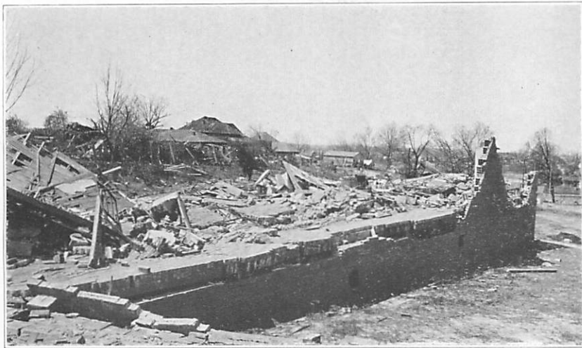
Figure 9.—The north wall of the south wing of the Church Street Grammar School, Tupelo, Miss., was blown southward flat across the small desks by the tornado of April 5, 1936.--Photographed April 13, 1936.
