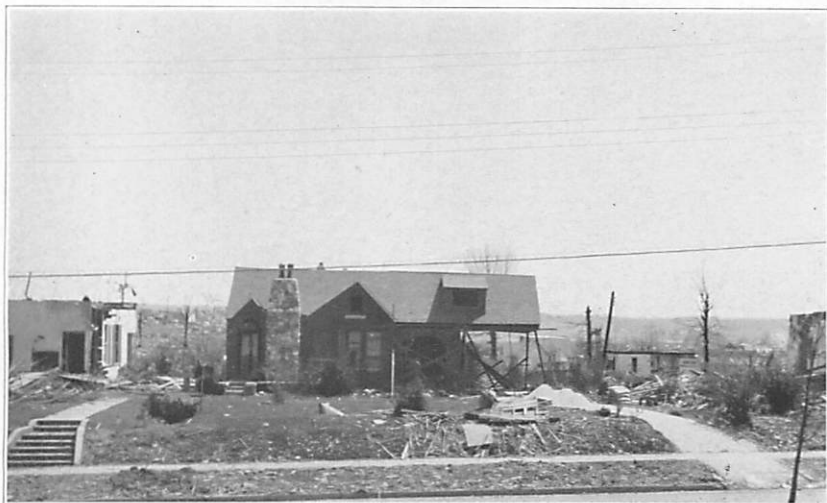
Figure 16.—Aside from a badly punctured roof, which had been replaced prior to the taking of this photograph on April 13, 1936, and shattered window panes, this brick veneer house of Mr. Vincent Carnaggio on Church Street opposite the Grammar School suffered only a battered down column and a dented rear wall, solely because it was excellently constructed with high grade cement mortar.
