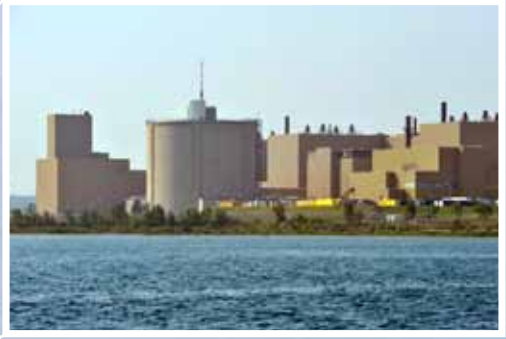
B03 | Bruce A Generating Station
