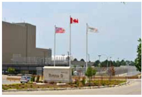
B05 | Bruce B Generating Station
