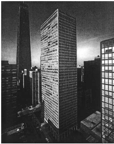
Figure 2 Chestnut-Dewitt Apartment Building, Chicago IL.
