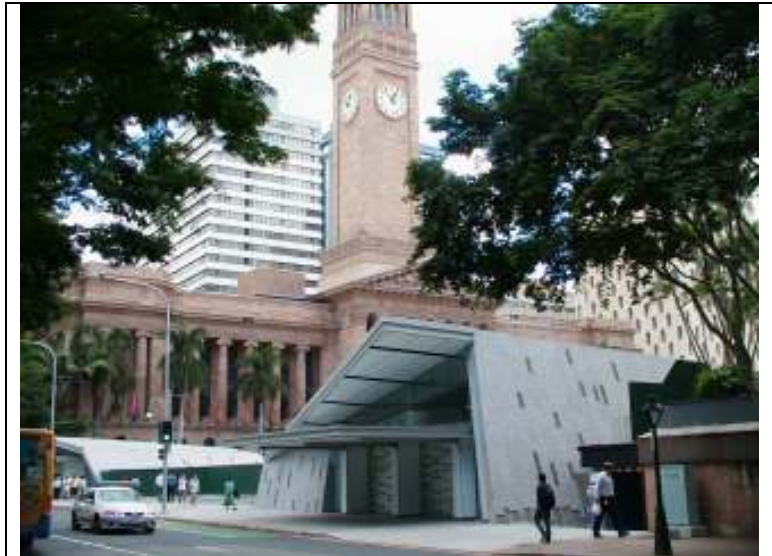
Entrance to King George Square Busway Station
