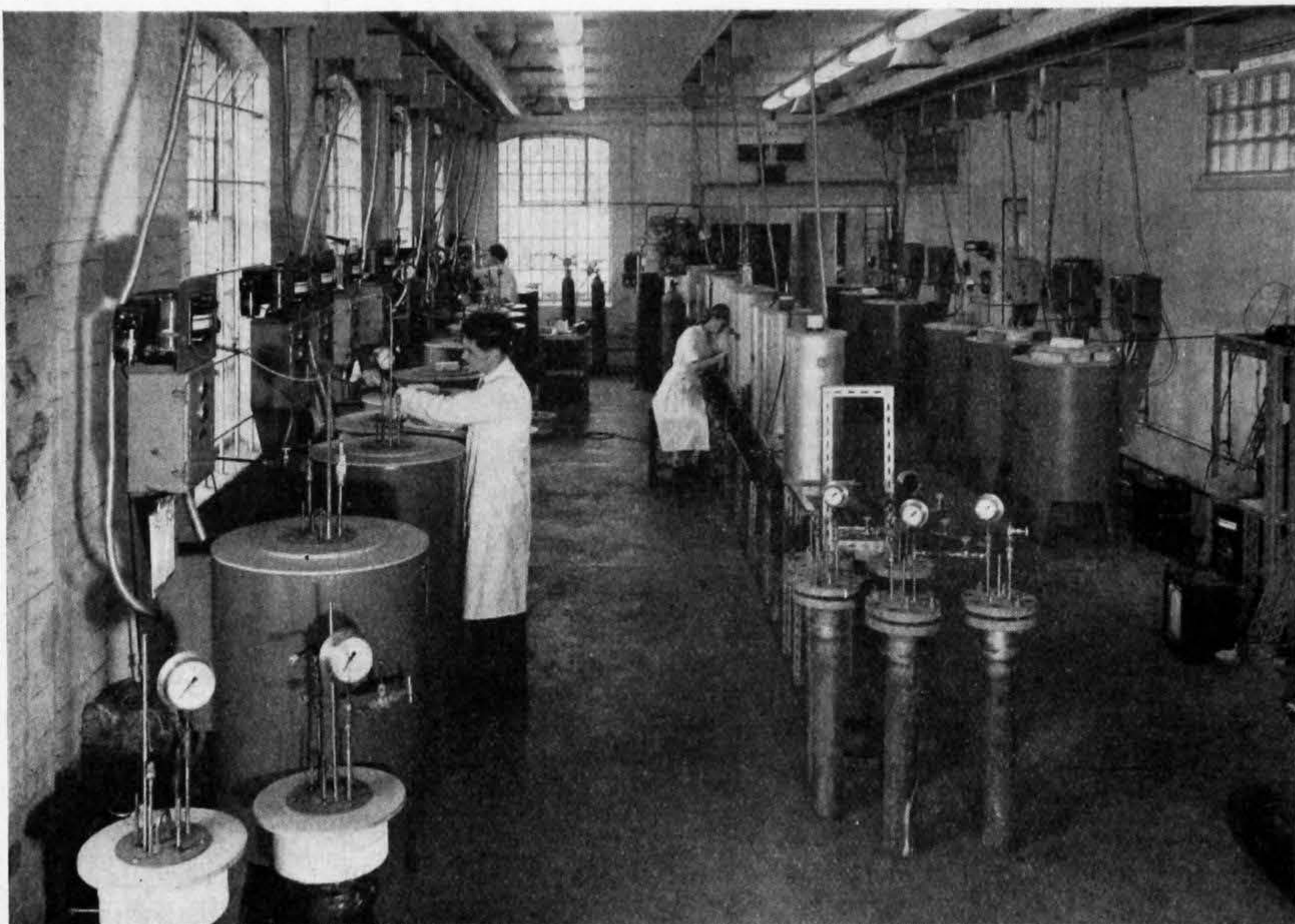
Fig. 6—Materials research laboratory for nuclear power development. The work done with the furnaces shown here includes compatibility, creep and corrosion tests in various atmospheres, including pure \text{CO}_2 and \text{CO}_2 contaminated with CO and moisture
