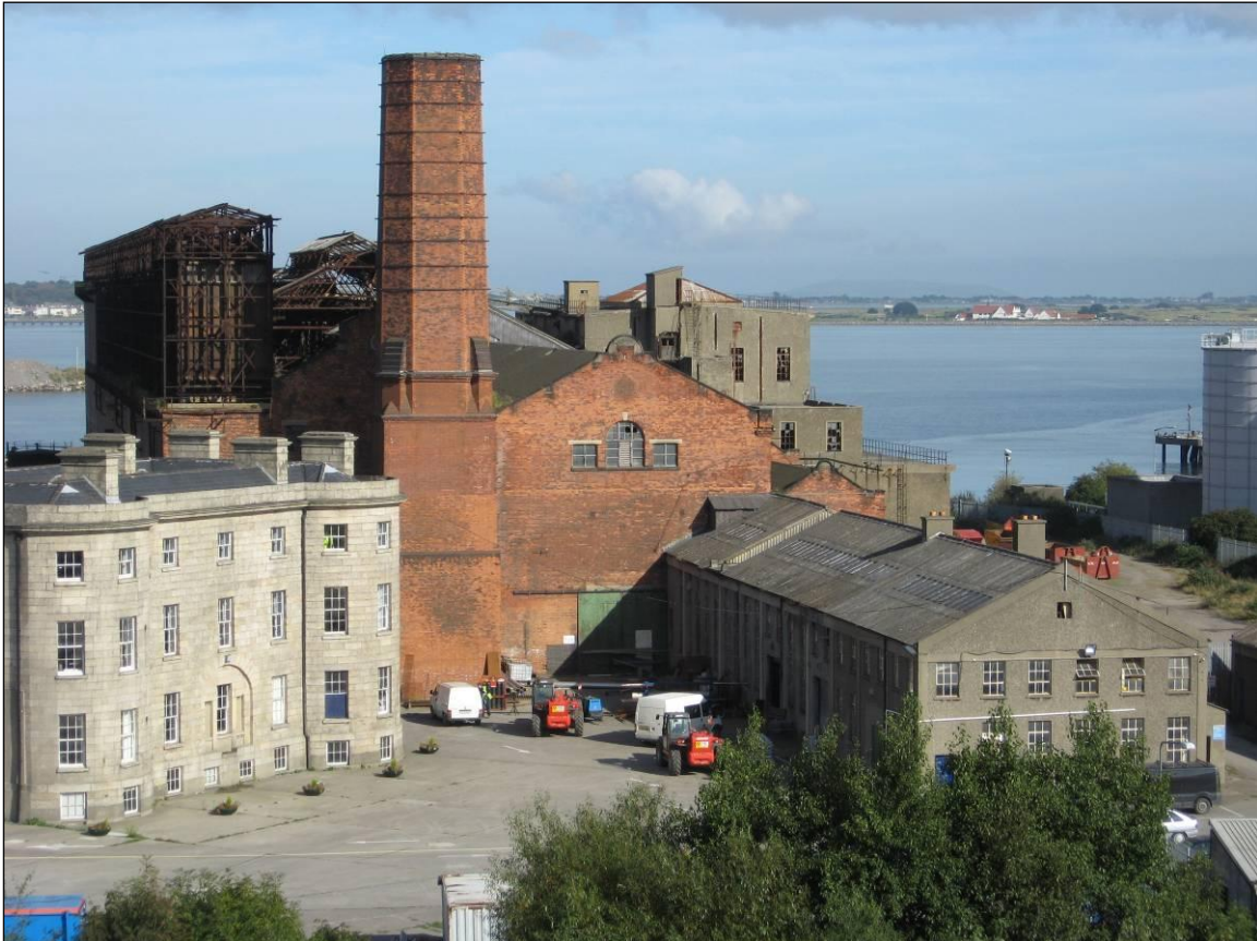
Pigeon House Power Station
