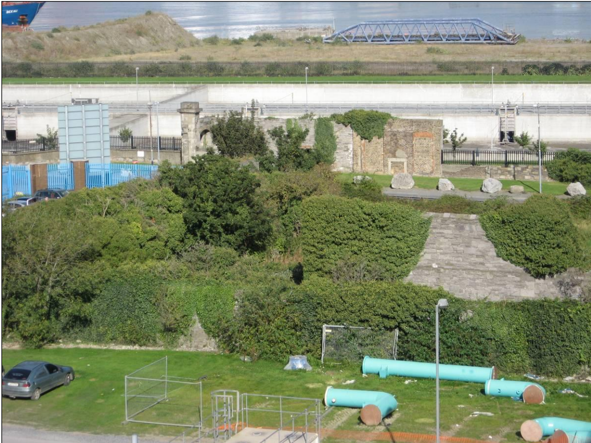
Upstanding remains of Pigeon House Fort
