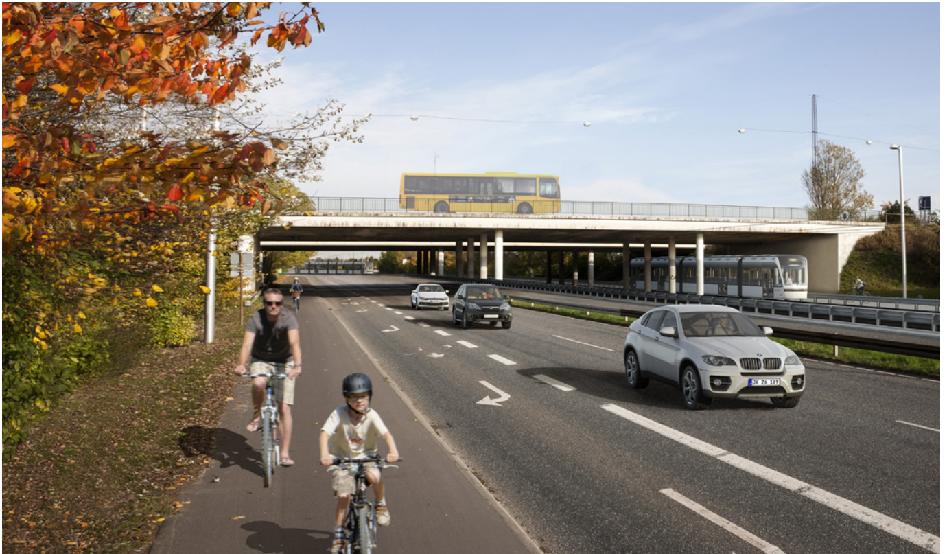
The entrance to the light rail's control and maintenance centre will be opposite Islevbro station at Rødovre.
