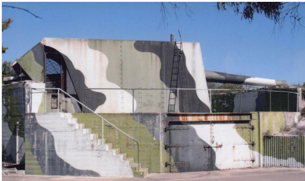
A fully enclosed and camouflaged 9.2-inch Mark 10 on a Mark 7 mounting at Robben Island Battery, off Cape Town, South Africa
