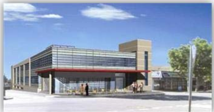
Council-owned Commercial building in St Marys (under construction)
