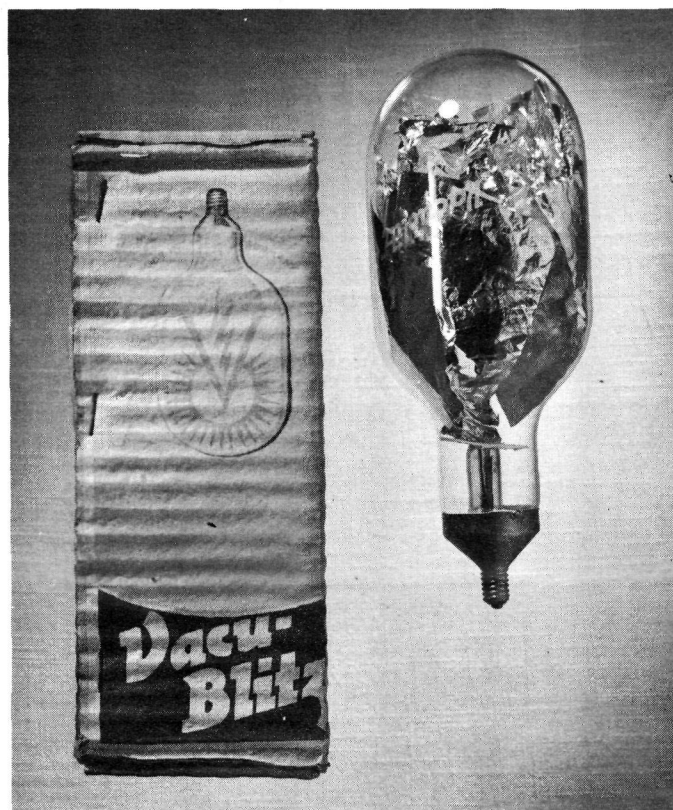
FIRST FLASH BULBS of 1929 were filled with aluminum foil.
