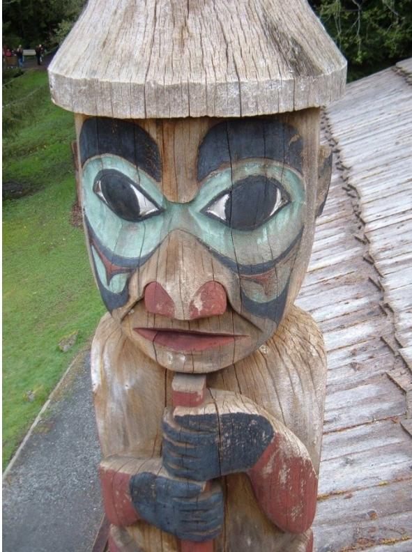
Surface cracks in hat and body
