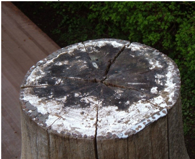
Split end grain of hat with remnants of lead cap
