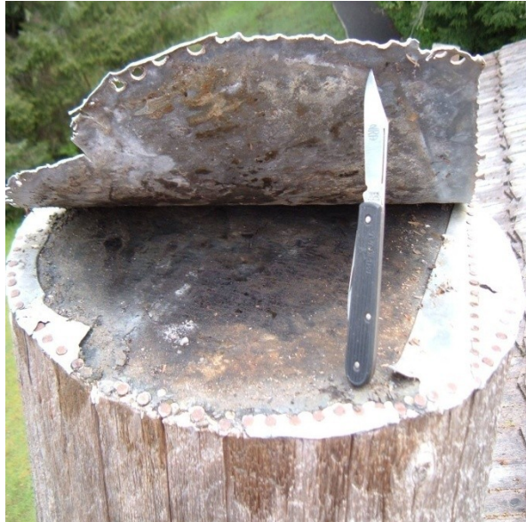
Revealing layer of felt paper
