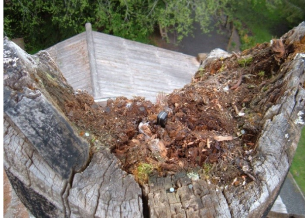
Spatula buried 12" into deteriorated head of Raven
