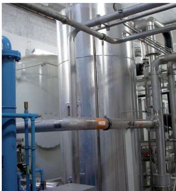
Photo 5. Column for hydrogen sulphide removal with activated carbon. After desulphurisation the gas enters a PSA-upgrading plant.
