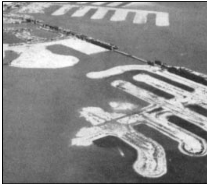
Dredging created miles of waterfront homes in Boca Ciega Bay in the 1950s and early 1960s. Above: Finger fills along the Treasure Island Causeway in 1956. Below: By 1976, fills in the bay off St. Petersburg Beach were filled with homes.
