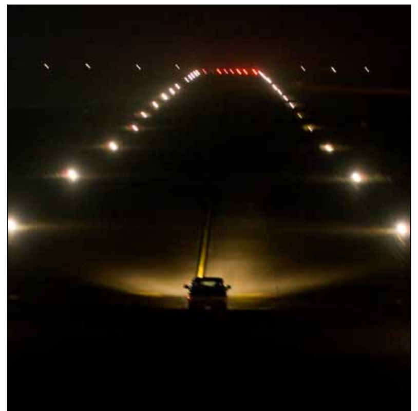
Eighth Civil Engineer Squadron Airmen inspect a runway lighting kit at Kunsan Air Base, Republic of Korea, Sept. 30, 2013. The kit allows Airmen to create an expeditionary runway with proper lighting for both night and daytime operations, even during a power shortage.
