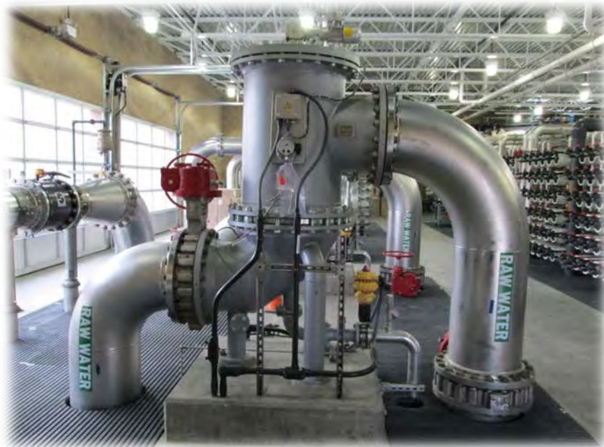
Figure 4.6 Automatic Backwashing Sand Separator
