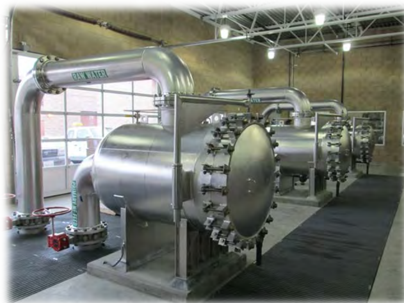
Figure 4.7 Cartridge Filter Housings
