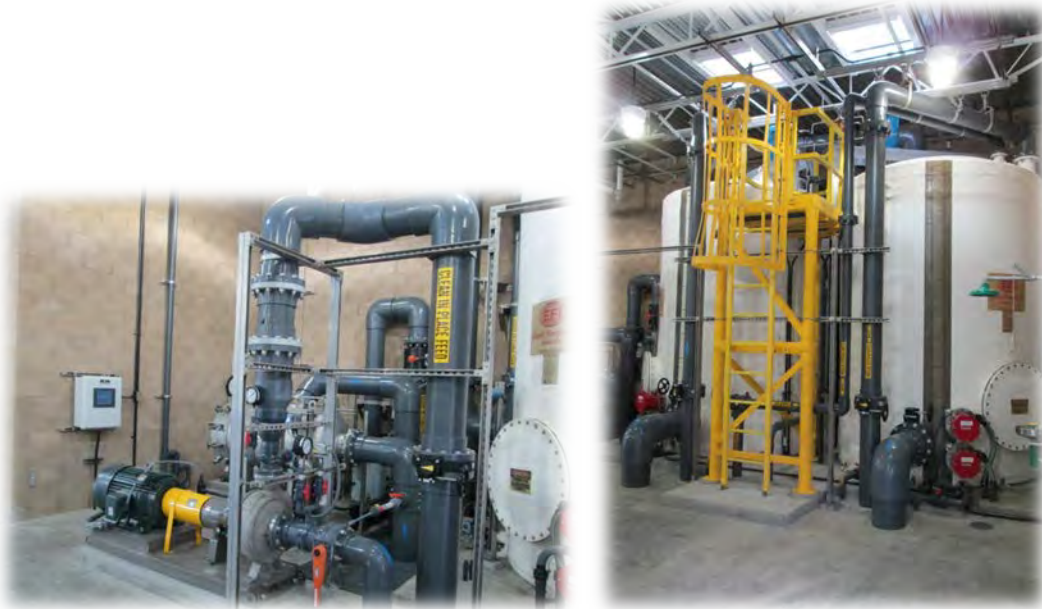
Figure 4.10 Typical CIP System
