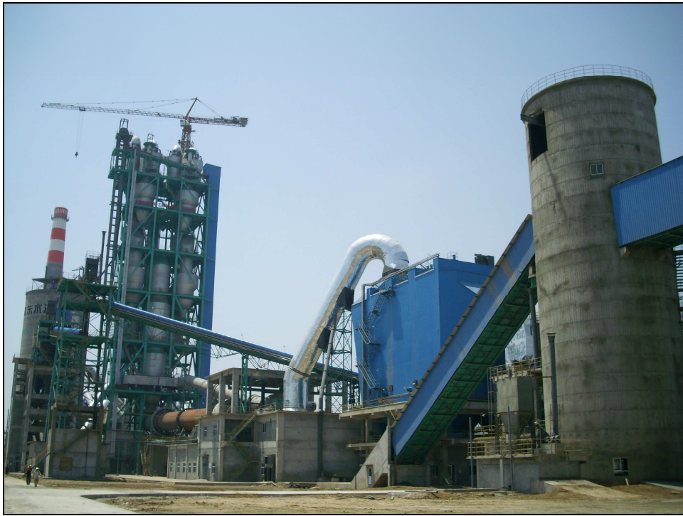
Abb. 24: Volan Zementwerk in Jining (China) 22
