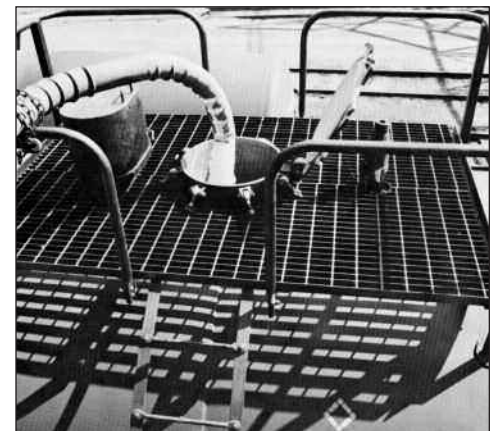
Loading caustic soda solution into tank car.
