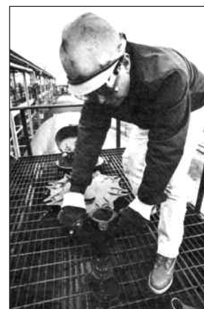
Testing internal valve handle.
