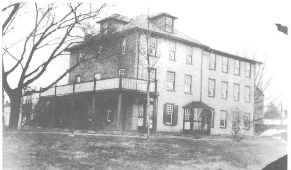
Walber's before additions
