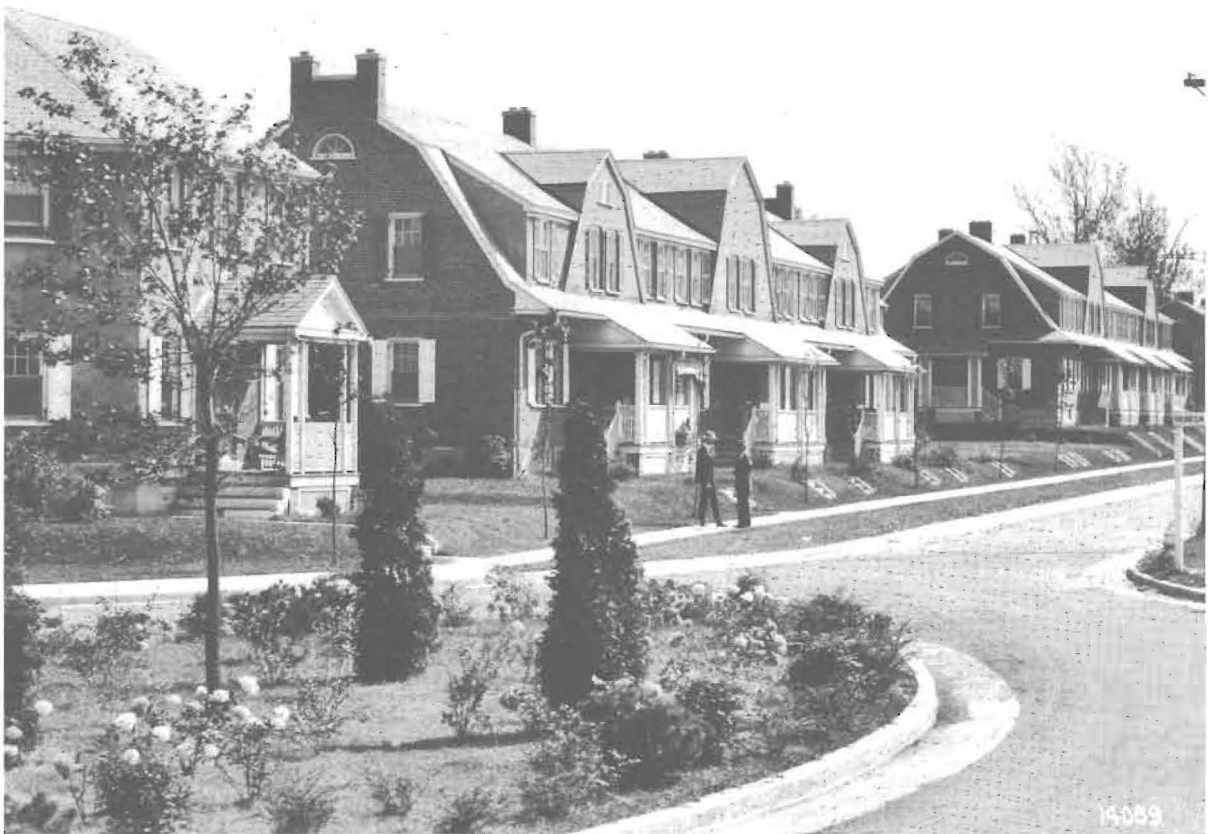
"Westinghouse Village" – this photo taken in the 1920's shows homes on Saude Avenue
