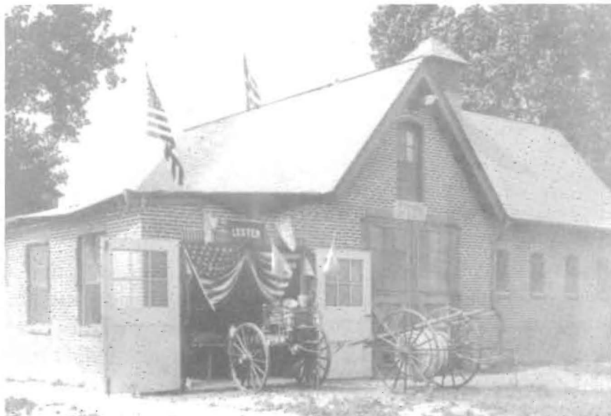
Lester Fire Company's first building
