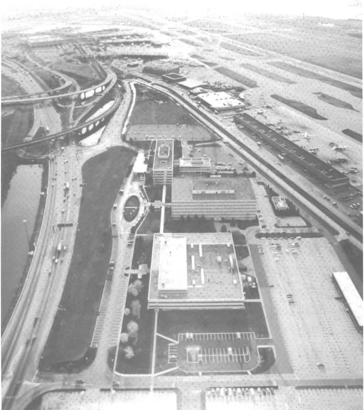
Aerial view of the Philadelphia International Airport (circa 1990).
