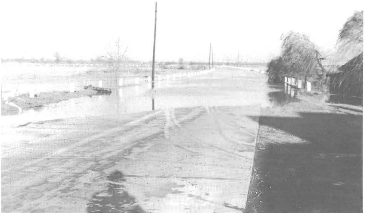
Island Road during the flood of 1932 (looking toward airport)
