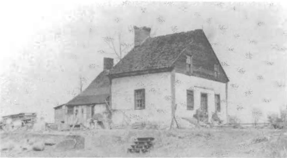
Old log cabin which was removed to make way for Westinghouse canal
