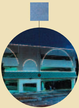
Form liner acid etch, water washed
