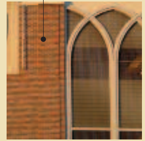
Light and medium blasts, granite veneer cast into panels
