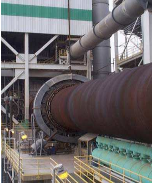
Picture 7. Cement Kiln. Source: [7].
