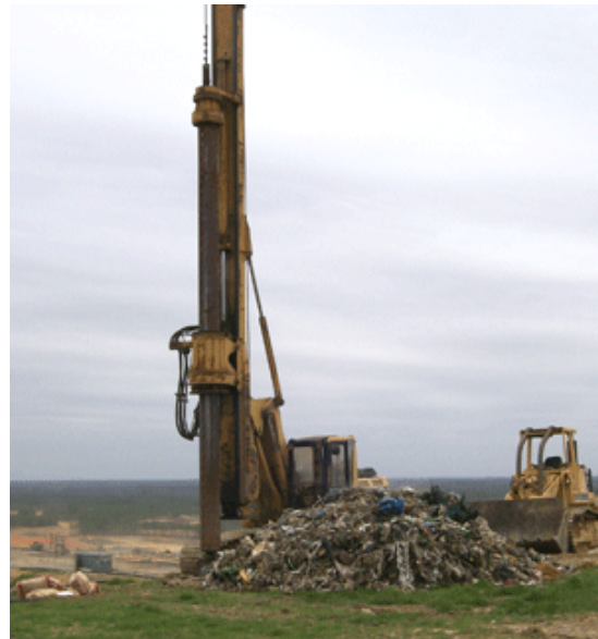
Picture 2. Wells drilling on reclaimed landfill. Source: http://www.kellettswell.com/drilling.html
