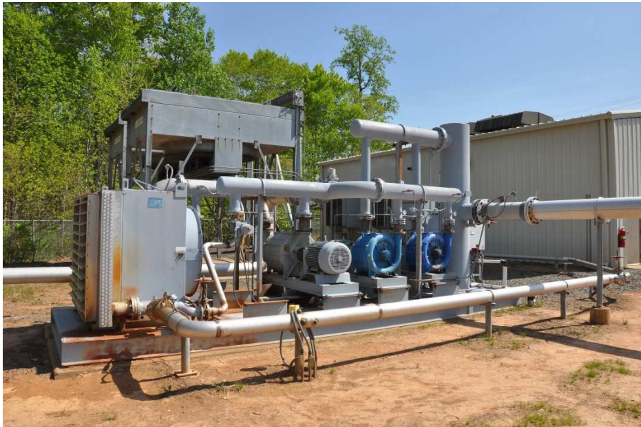
Picture 4. Gas collection system on Prince William County landfill, USA. Source: INiG photo.
