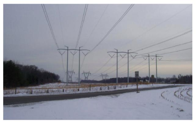
500 kVAC US transmission corridor Multi GW DC transmission can be trenched in parallel
