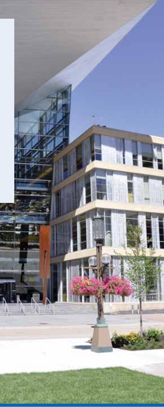
Pictured right: Hennepin County Library - Minneapolis Central
