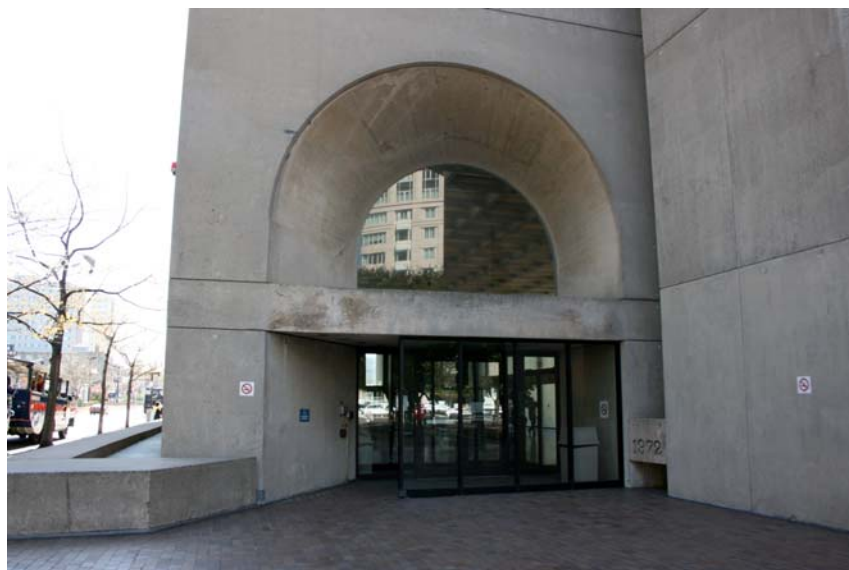
Figure 13. Administration Building: Main entrance facing Belvidere Street. (Photograph by Wendy Frontiero)
