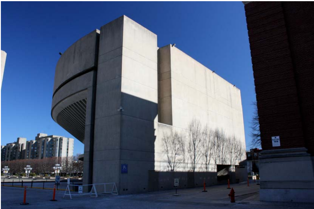
Figure 15. Sunday School Building: Service alley elevation. (Photograph by Wendy Frontiero)
