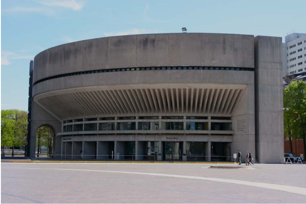
Figure 14. Sunday School Building: Plaza façade. (Photograph by Wendy Frontiero)
