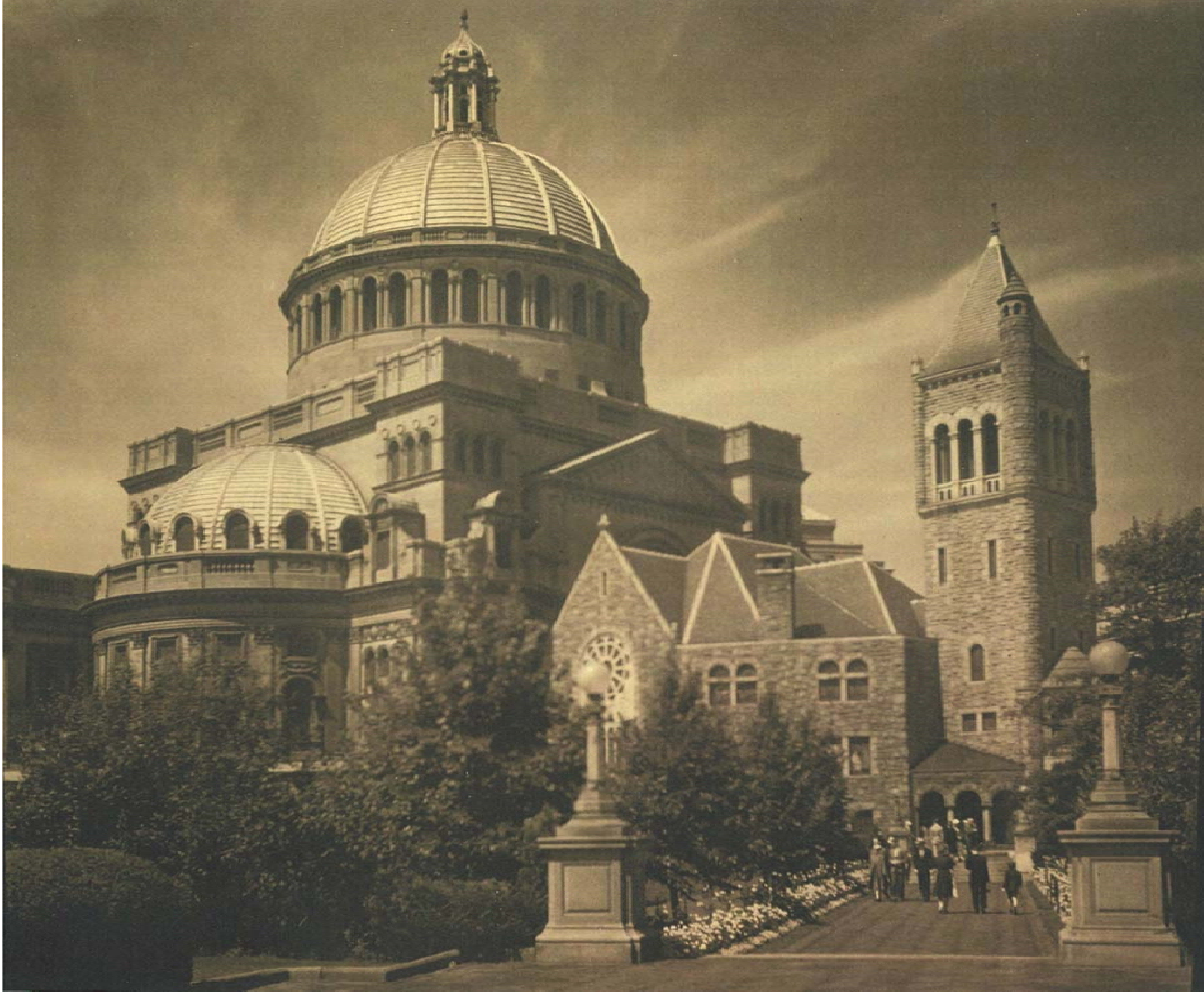
Figure 27. Historic view (mid-20 th century) of The Mother Church Extension, Original Mother Church, and Church Park. (Photograph courtesy of Robert A. Herlinger)
