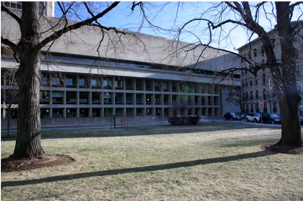
Figure 11. Church Colonnade Building: Back elevation. (Photograph by Wendy Frontiero)
