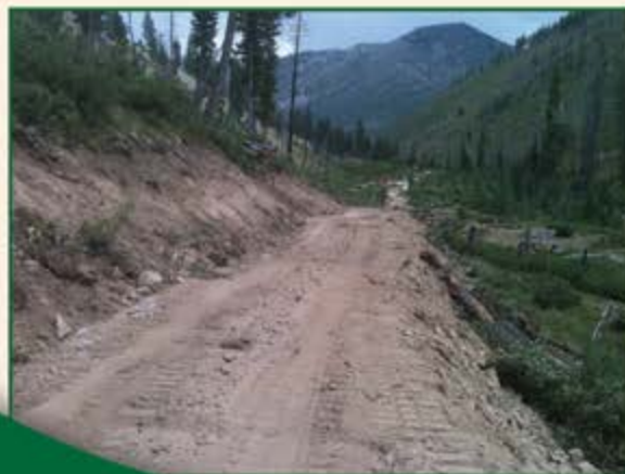
Left: Graham Road after crews repair washout.
