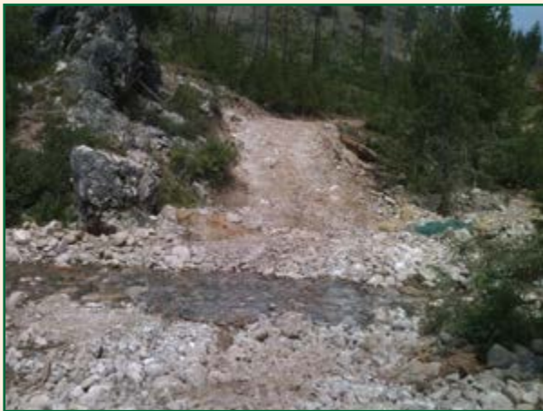
Above: Section of Graham Road washed out in 2010 from flooding.
