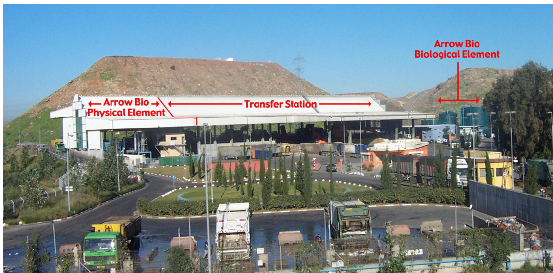
FIGURE 1. THE ARROWBIO PLANT AT THE TEL AVIV, ISRAEL, TRANSFER STATION. THE FRONT-END PHYSICAL SEPARATION/PREPARATION STAGE OF THE PLANT IS UNDER THE ROOF AT THE LEFT, AND THE BACK-END BIOLOGICAL STAGE IS BEYOND THE ROOF AT THE RIGHT. THE BACKGROUND IS THE HIRIYA DUMP, NOW CLOSED AND BEING REMEDIATED AS PART OF AYALON PARK.
