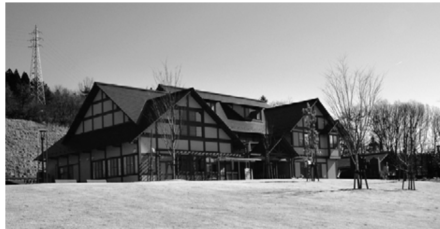
Katsura River Wellness Park (Satoyama Exchange Center)
