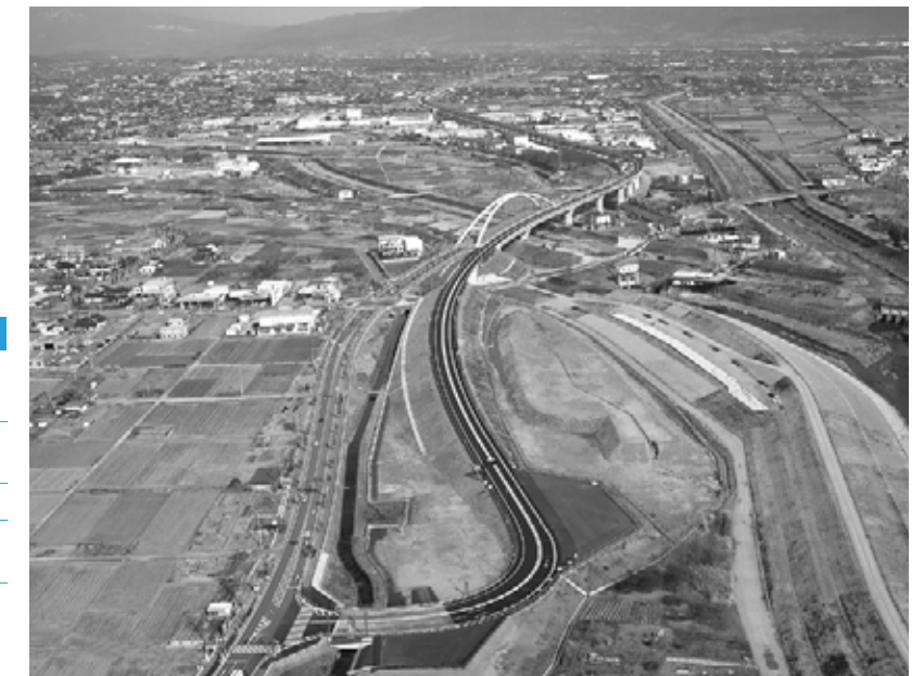
The Masuho Interchange of the Chubu-Odan Expressway
