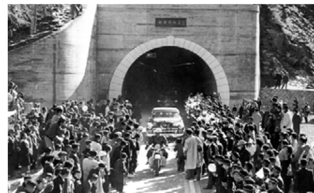
Opening of the Shin-Sasago Tunnel
