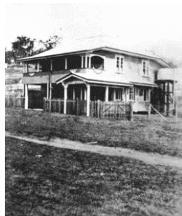
Queensland Ambulance Station in Appel Street, Canungra, c.1917 Source: John Oxley Library, State Library of Queensland, Image no: 111867.
