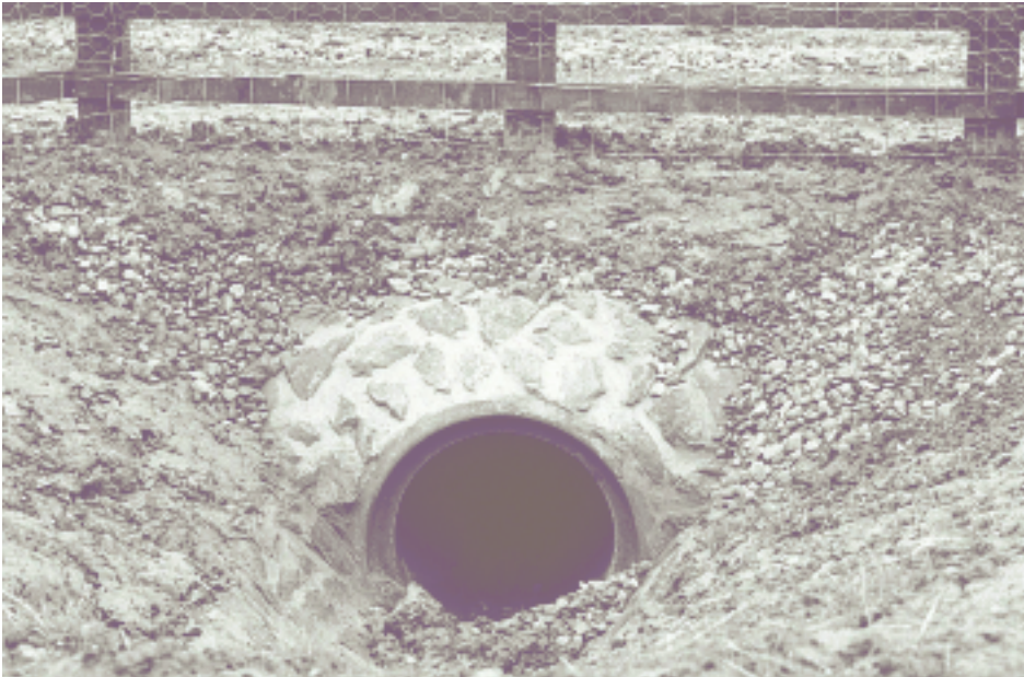
A completed badger tunnel with associated fencing
