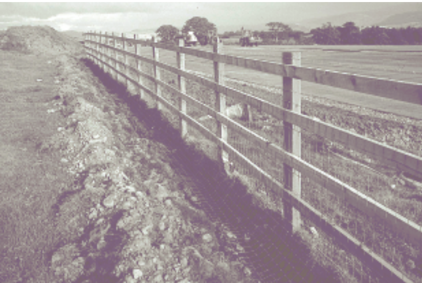
BADGER RESISTANT MESH ATTACHED TO A TIMBER & FOUR RAIL FENCE
