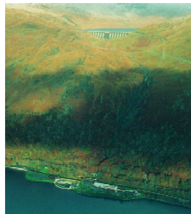
■ Cruachan upper reservoir and the station offices far below at Loch Awe
