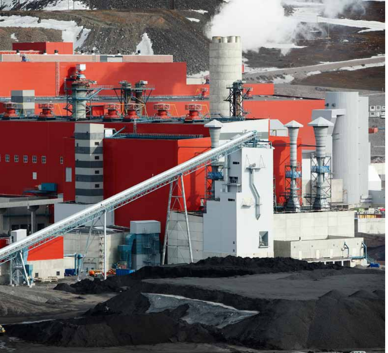
LKAB's newest pelletising plant, KK4 in Kiruna, is counted among the pelletising plants with the world's lowest emissions. Thanks to an investment of SEK 700 million, Bandugnsverket, Malmberget's oldest pelletising plant, is soon also counted among these clean pelletising plants.
