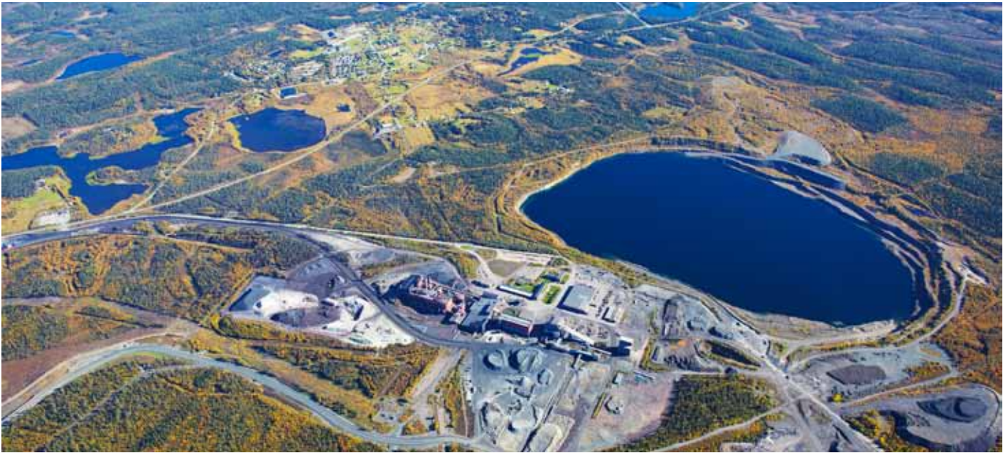
Open-pit mine Leveäniemi opened in 1964 but was closed in 1983 for market reasons. LKAB now plans to reopen it as one of three new mines in the Svappavaara field. The other two are Gruvberget and Mertainen.
