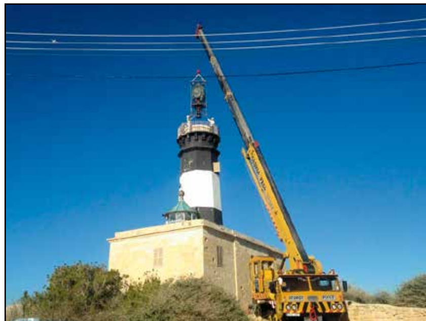
The mechanism and housing being hoisted into place
