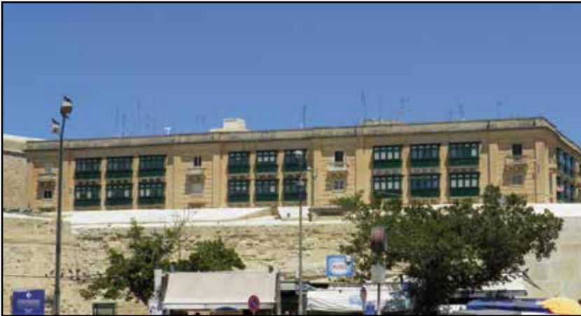
Retrofitting of the social housing façades
