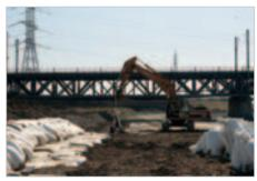
Placing of soil filled Secutex® scour protection sandcontainers
