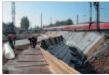
Secuarid® geogrid installation in the embankment slope
