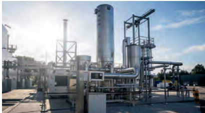
The methanation reactor at the Audi e-gas plant in Werlte enables synthetic natural gas to be produced.
