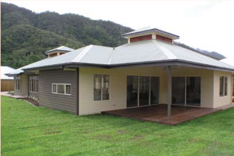
Sustainable Home Redlynch Valley showing use of light colours and large openings for cross ventilation.
