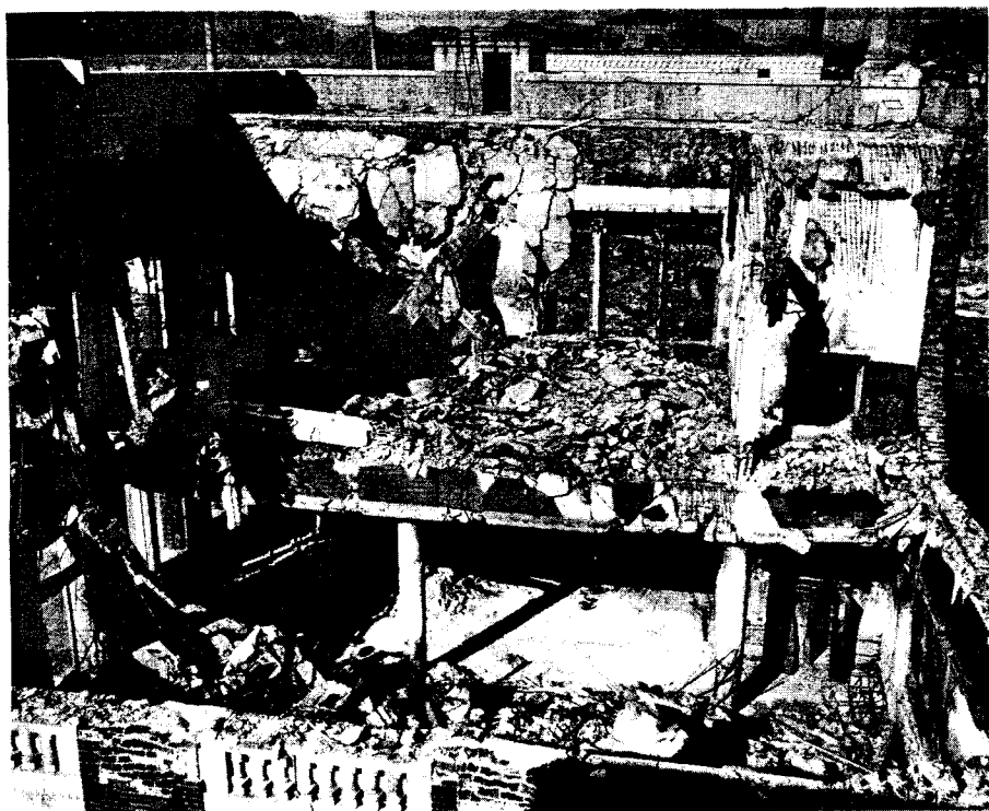
Figure 5.23. Reinforced-concrete building showing collapsed roof and floor slabs (0.10 mile from ground zero at Nagasaki).
