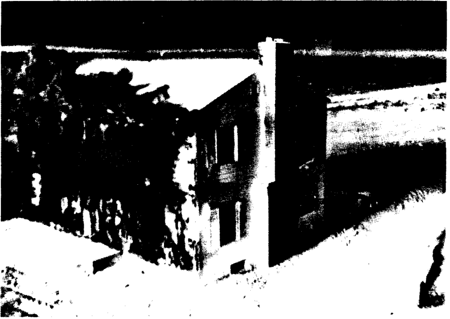
Figure 7.28a. Thermal effects on wood-frame house 1 second after explosion (about 25 \text{ cal/cm}^2 ).
