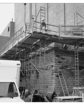
Any place where tools, debris, or materials are piled higher than the toeboard, a screen must be built from the toeboard to the top of the guardrail to prevent items from falling.
