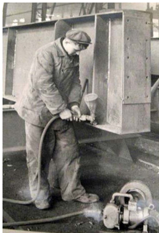
Fig. 10. Semiautomatic submerged arc welding (EWI archive photograph)
