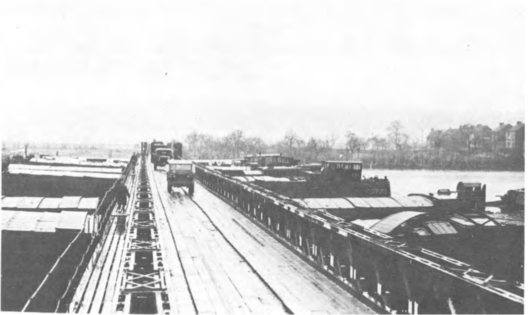
HIGHWAY BRIDGE OVER THE MEUSE RIVER, built with Bailey bridge spans over river barges.
