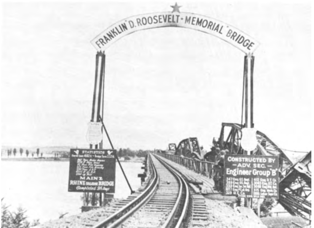
SINGLE-TRACK RAILROAD BRIDGE AT MAINZ constructed by Engineer Group B.
