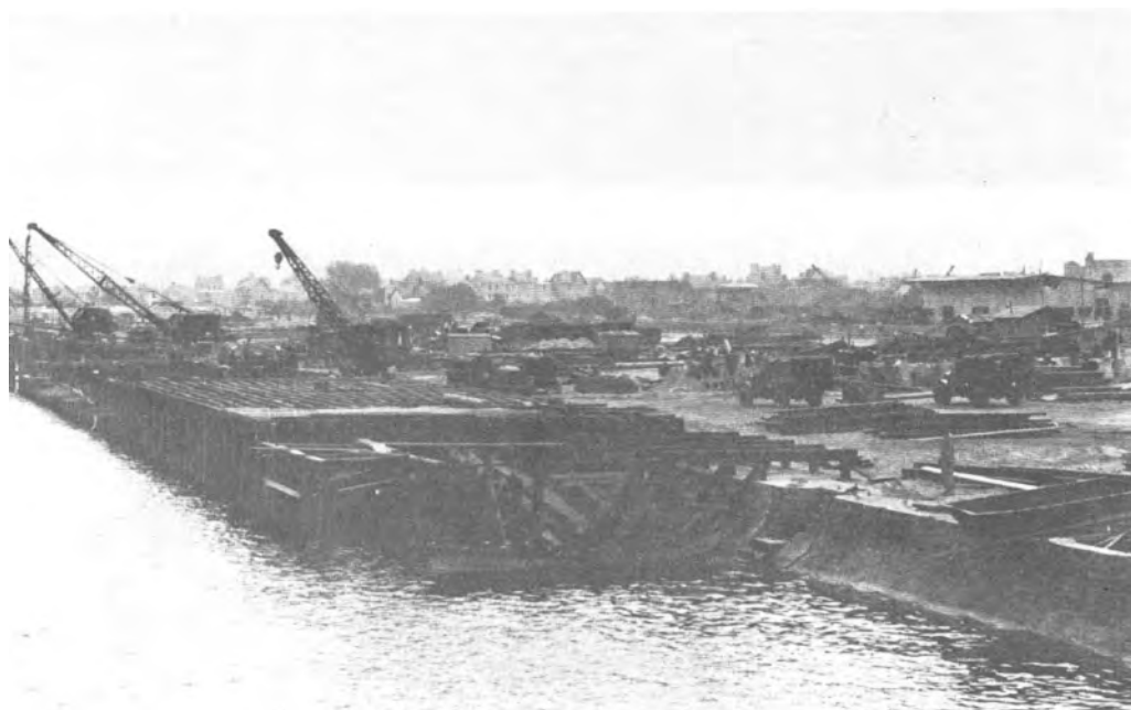
MARGINAL WHARF CONSTRUCTION along the Terre Plein, Cherbourg, 24 July 1944.
