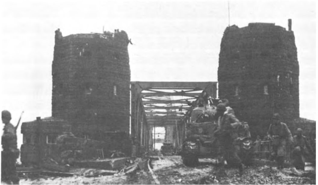
LUDENDORFF RAILWAY BRIDGE over the Rhine River at Remagen captured by men of the 9th Armored Division.
