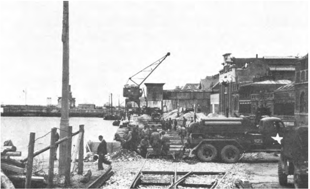
LAYING RAILWAY TRACKS for reception of supplies, Bassin à Flot, Cherbourg, 13 July 1944.
