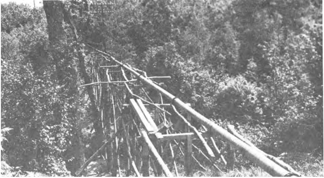
PORTION OF THE MAJOR PIPELINE passing over an improvised trestle bridge.
