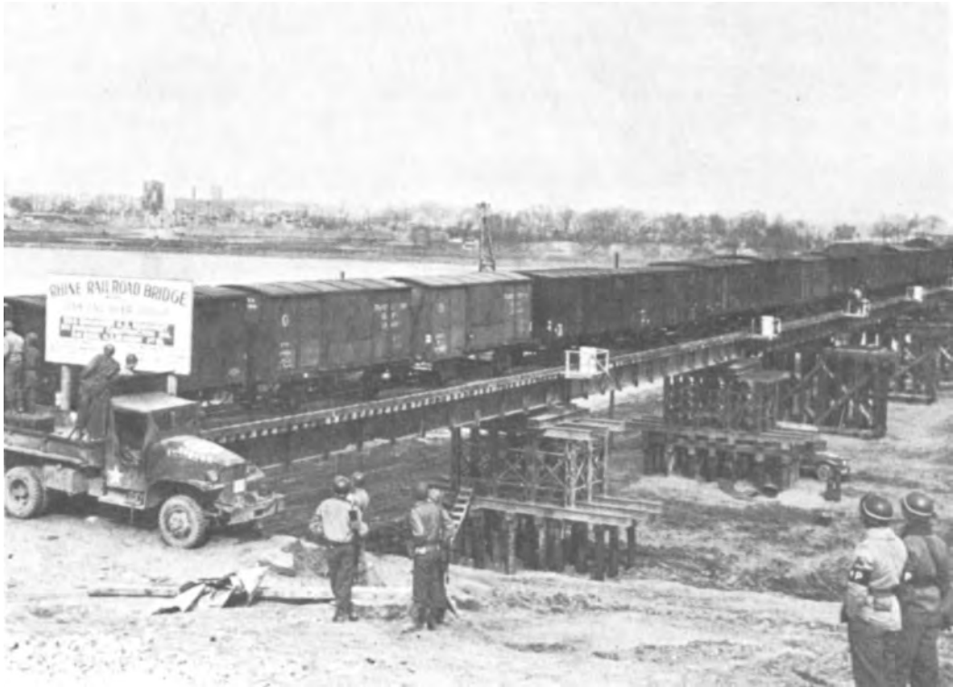
BRIDGE ACROSS THE RHINE AT WESEL constructed by 1056th PC&R Group.
