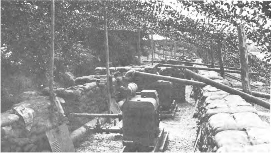
CAMOUFLAGED PUMPING STATION along the pipeline from Cherbourg.
