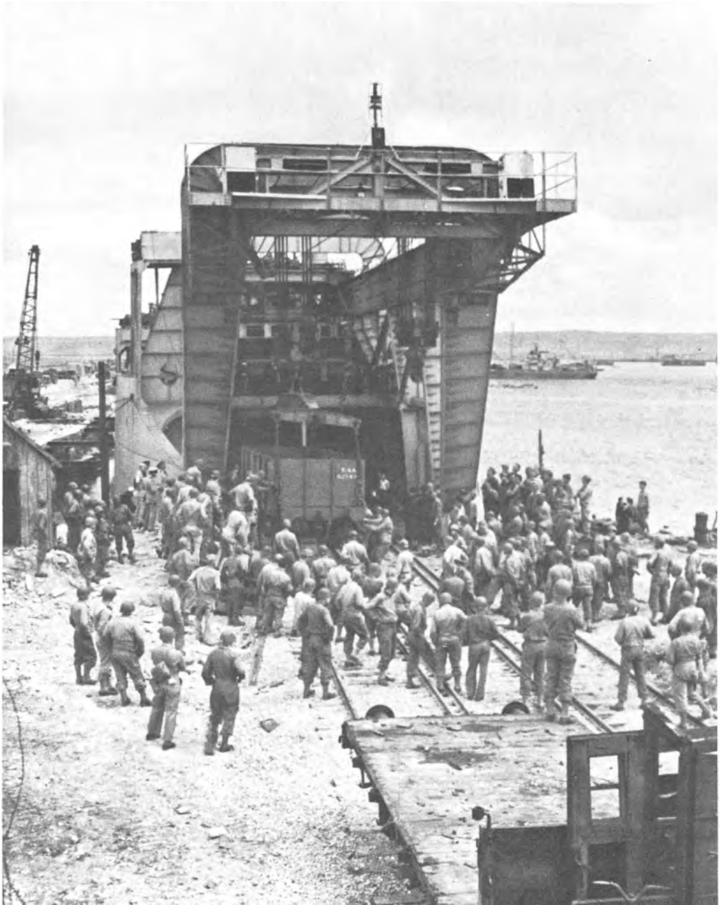
SEATRIN UNLOADING A GONDOLA onto rail lines laid to the water's edge, Cherbourg, August 1944.
