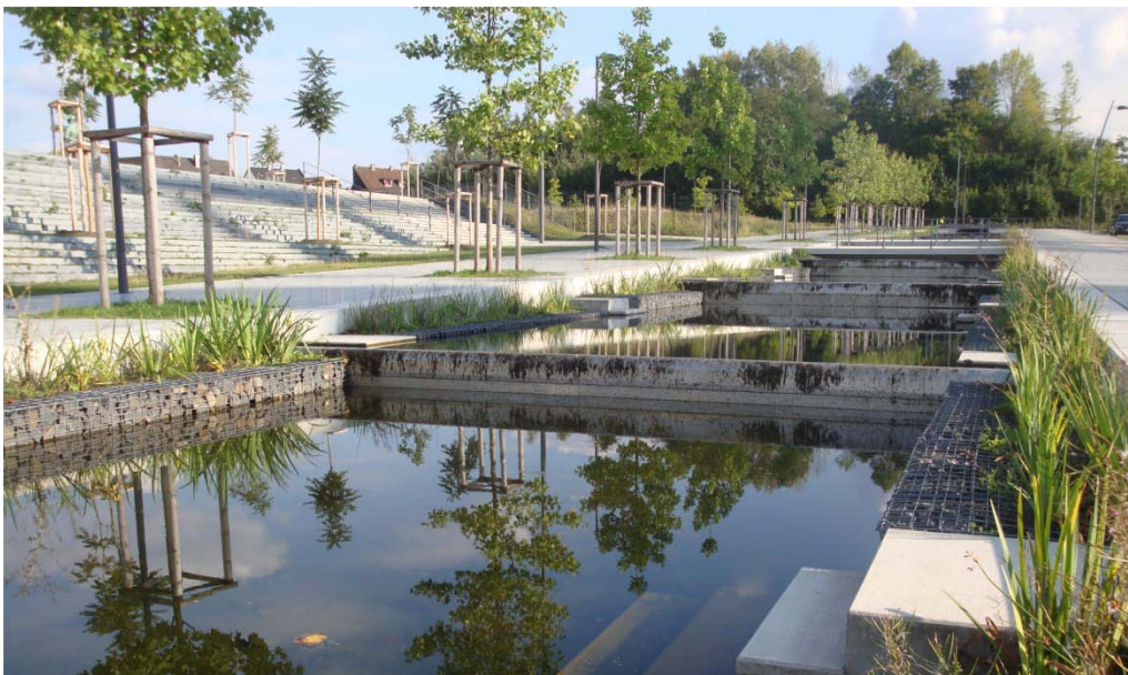
Image: The open grounds of the PHOENIX West blast furnace facility is transformed into a modern services location, surrounded by an extensive landscape park. Technical necessities (development, retention, building management) and ecological requirements are integrated and the banked design forms the basis for the new potential landscape.
