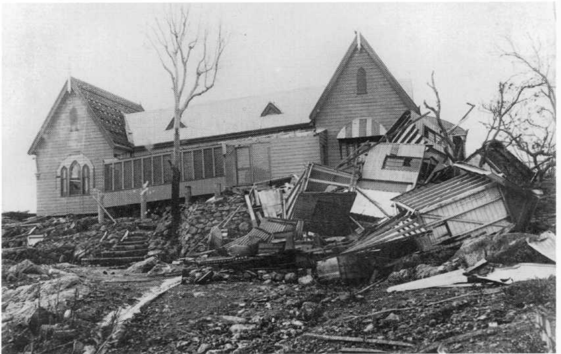
St James Rectory, Townsville, after cyclone Leonta , 1903. Back view showing the remains of the kitchen and outbuilding.
