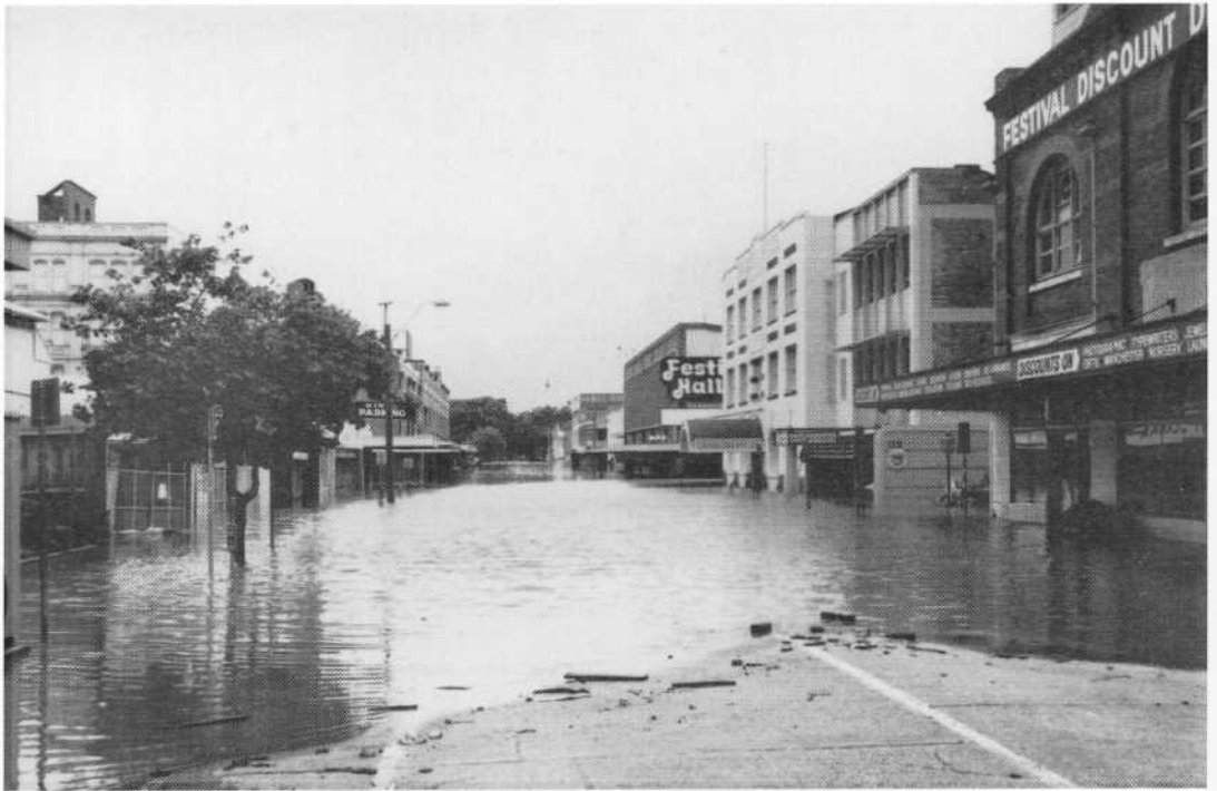
Flooding, Albert Street, Brisbane, 1974.
