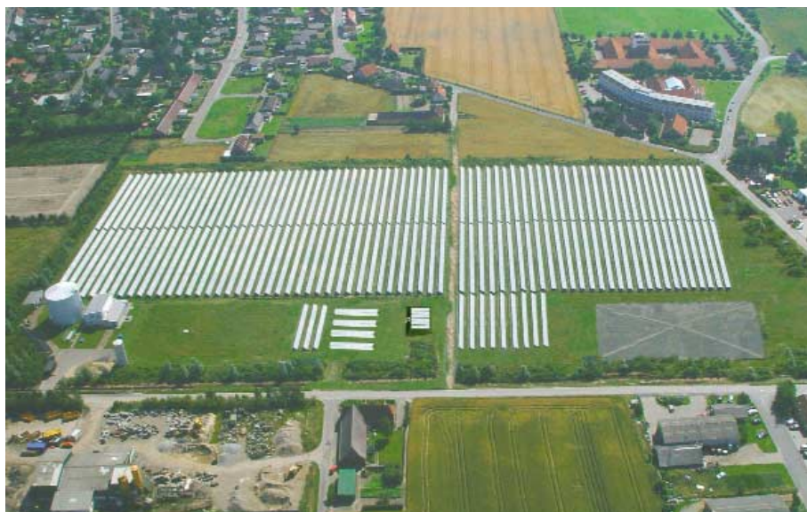
Photo: Marstal District Heating Company
