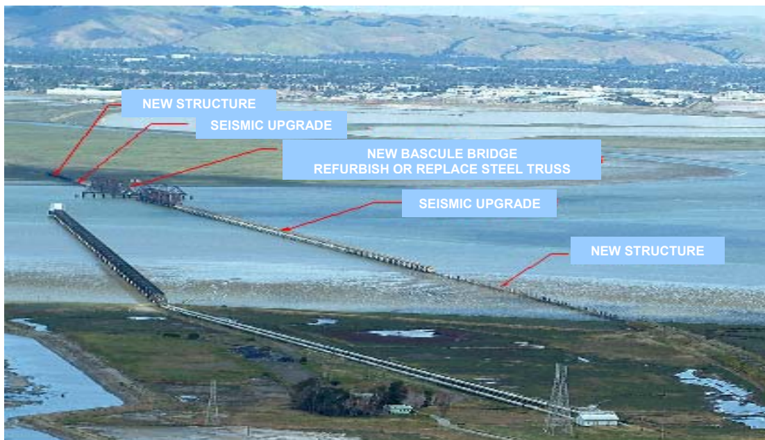
Figure 6: Main Elements of the Existing Dumbarton Bridge
