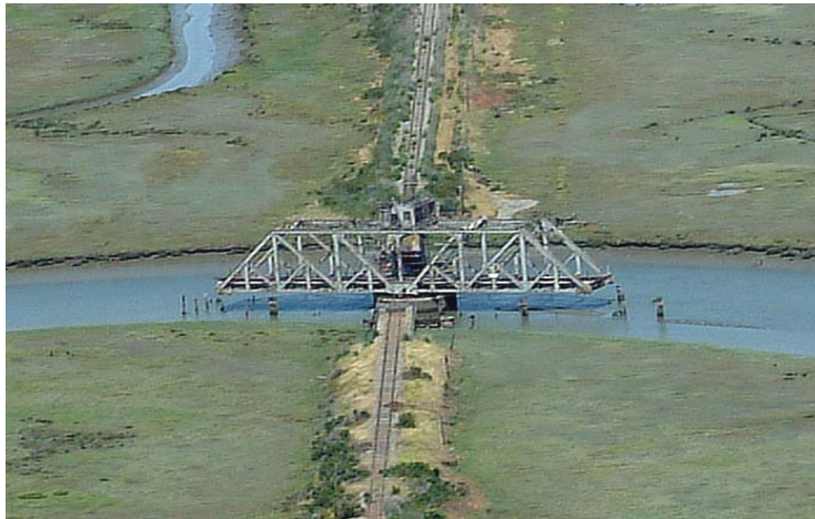
Figure 8: Existing Newark Slough Swing Bridge
